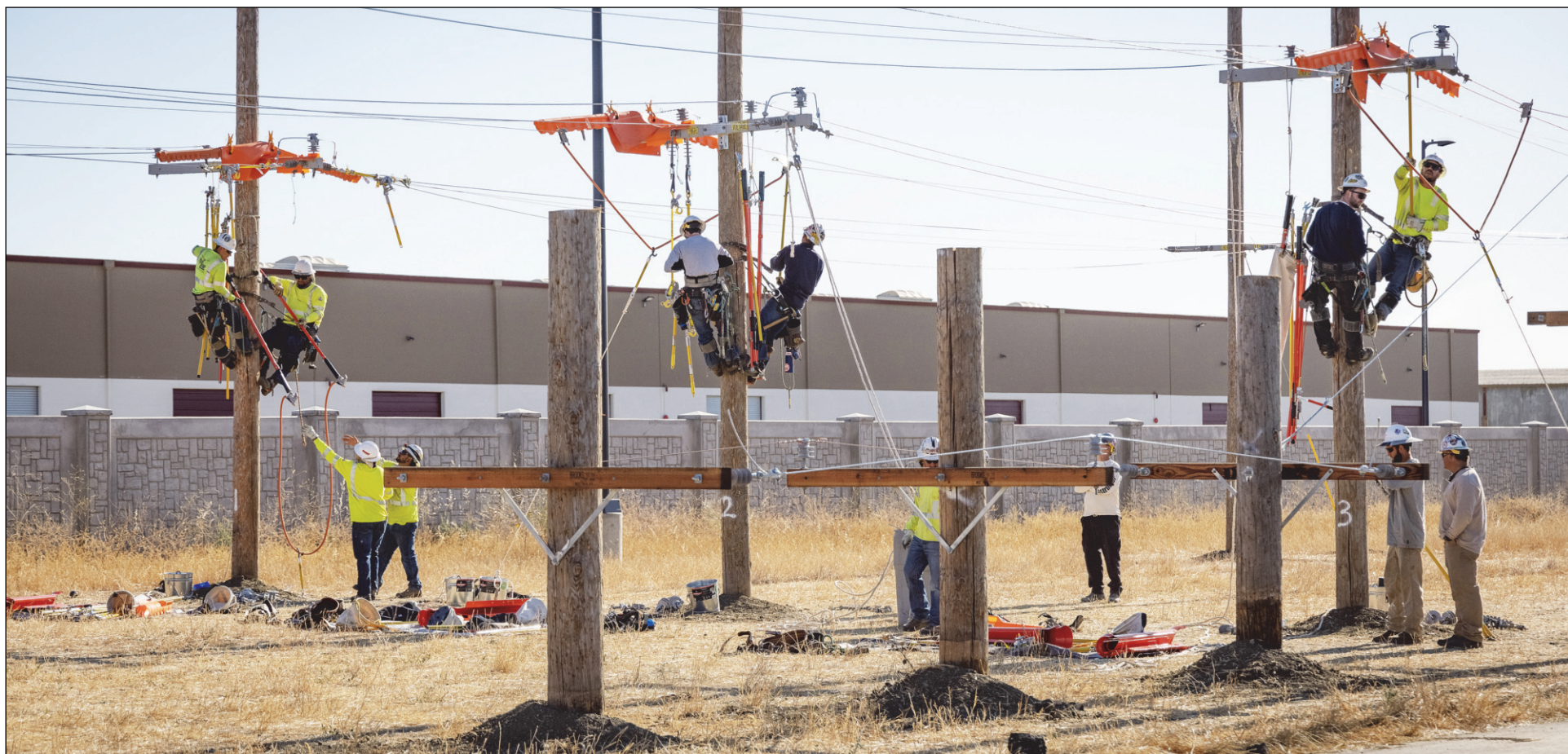
Apprentices get hot stick training at the JATC in Woodland
