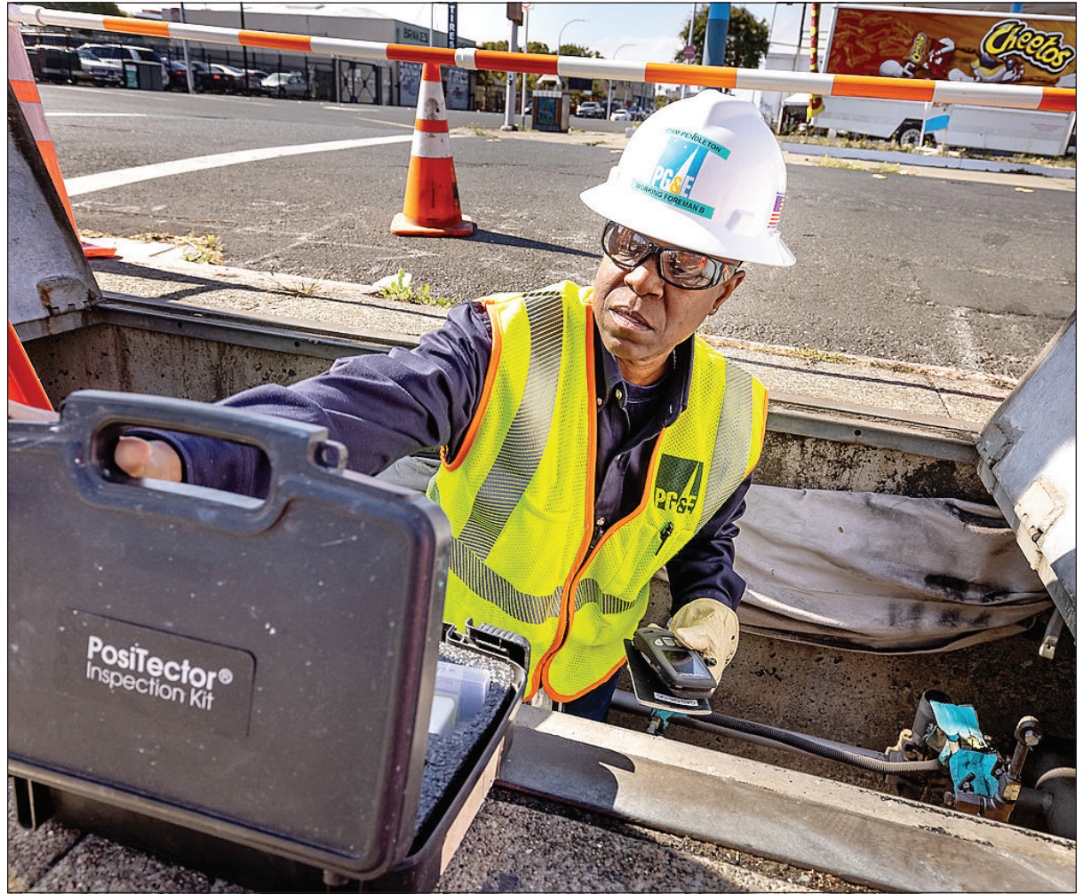
Working Foreman B Pam Pendleton
