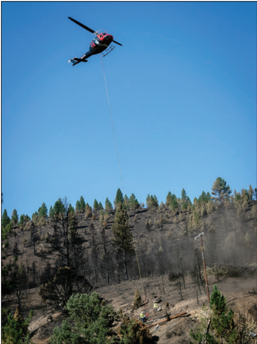
A Wasatch crew flies in a pole using a helicopter.
