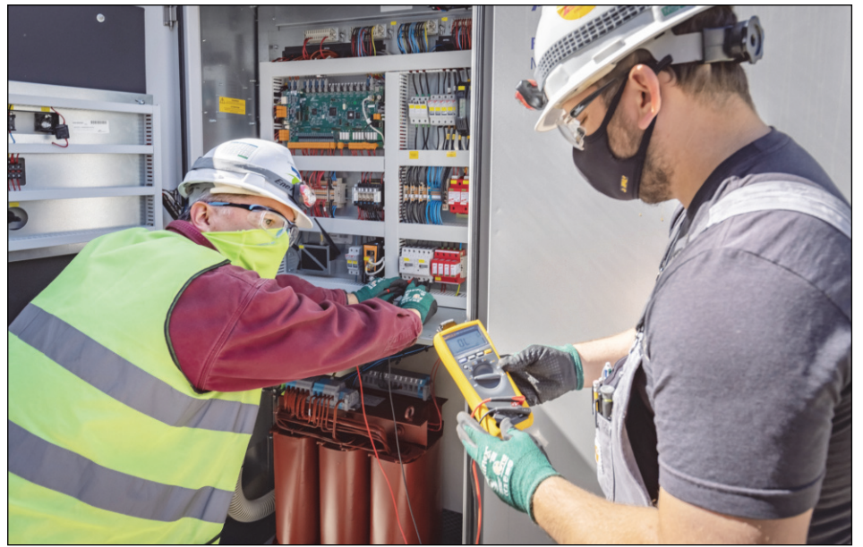
Nicholas Covello (right) and Jaime Rivera check voltage on the inverters.
