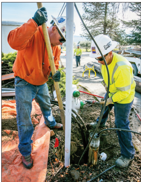
Derek Holt, left and Carlos Torres dig a hole for a new power pole.
