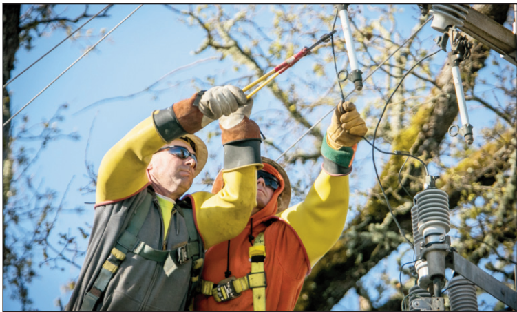
Kevin Guy (left) and Derek Holt change out a power pole.
