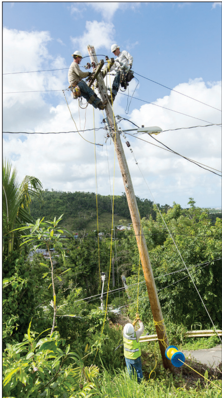
Rich Hall and crew replaced a cross arm and pulled new wire from down the hill.
