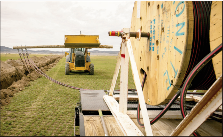
Chad Bliss lays power cables in a trench.
