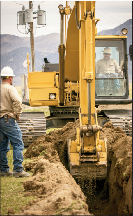
Bill Baumann digs a trench for underground power lines.
