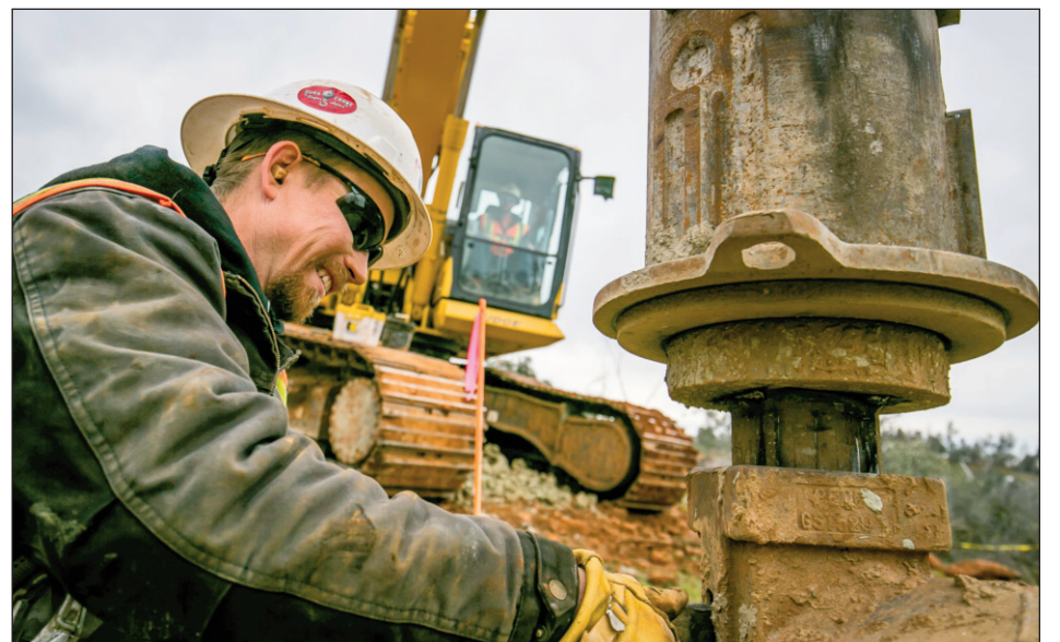
IBEW 1245 groundman Bobby Fox changes the drill bit as he drills holes for new poles.
