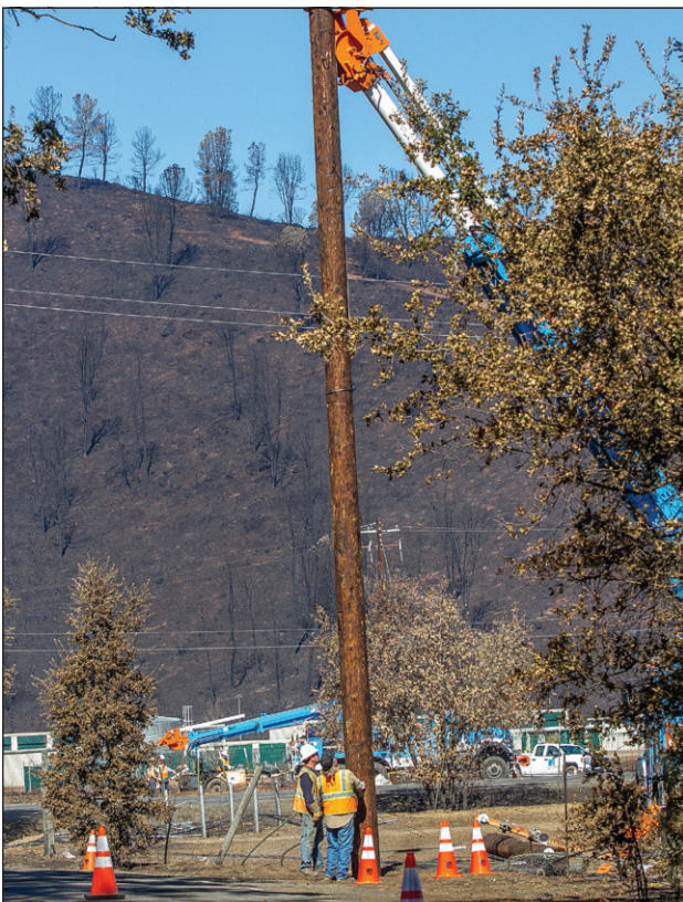
PG&E apprentice Dustin Trimble cleans the drill after digging a new hole for the replacement pole.
