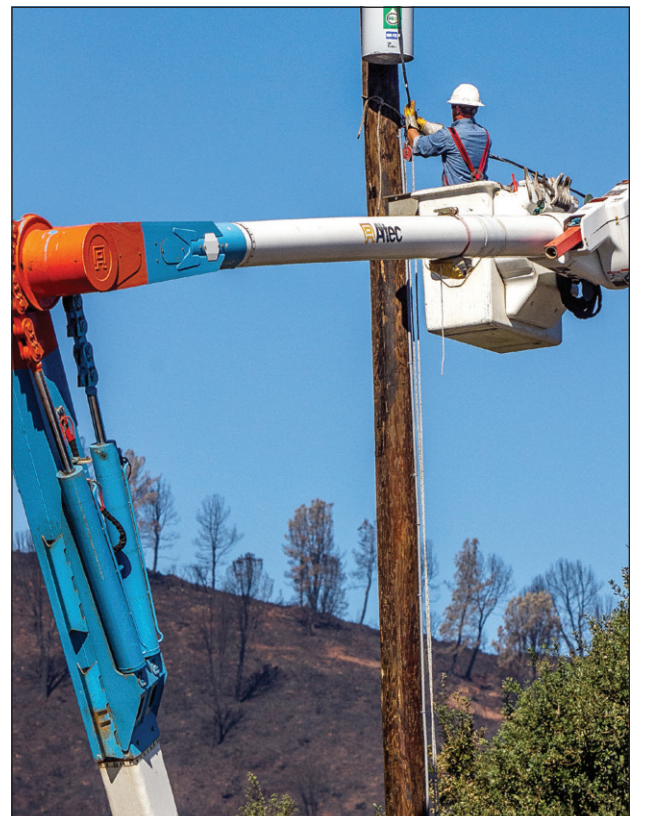
Lineman Jake Southard rolls out wire for connection to the new pole.
