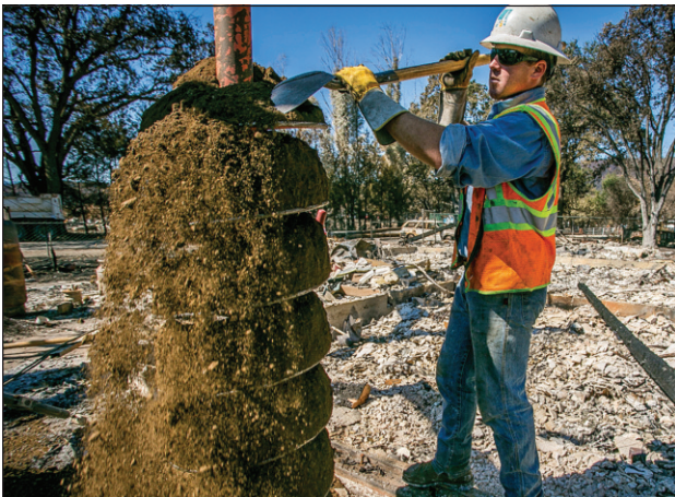
PG&E apprentice Dustin Trimble cleans the drill after digging a new hole for the replacement pole.
