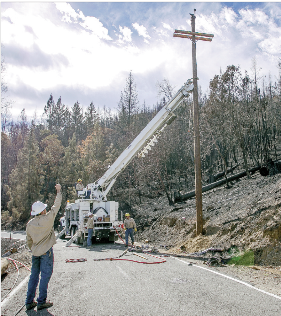
The Roseville crew works together to set a pole.
