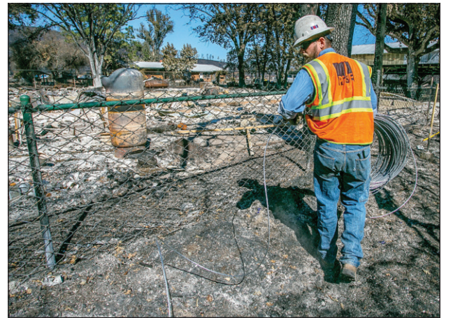
Lineman Jake Southard rolls out wire for connection to the new pole.
