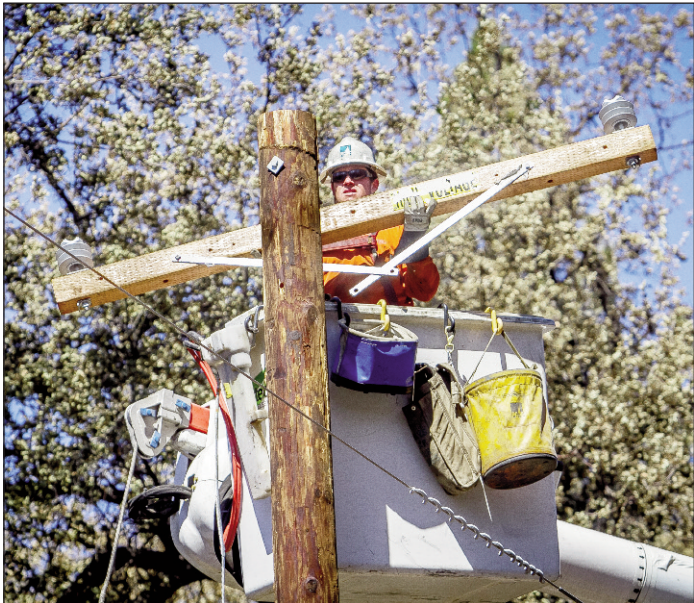
PG&E lineman Josh Ramos attaches a cross arm to a pole.
