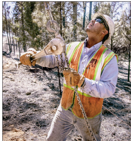
PG&E lineman Joe Menor tightens a guy wire on a new pole.
