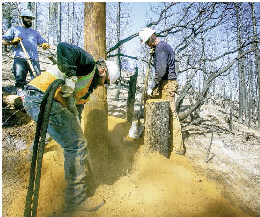
PG&E apprentices Matt Atkins (left), pre-apprentice Kyle Gustason (middle), and Brian Hinckle set a pole on the side of a mountain.
