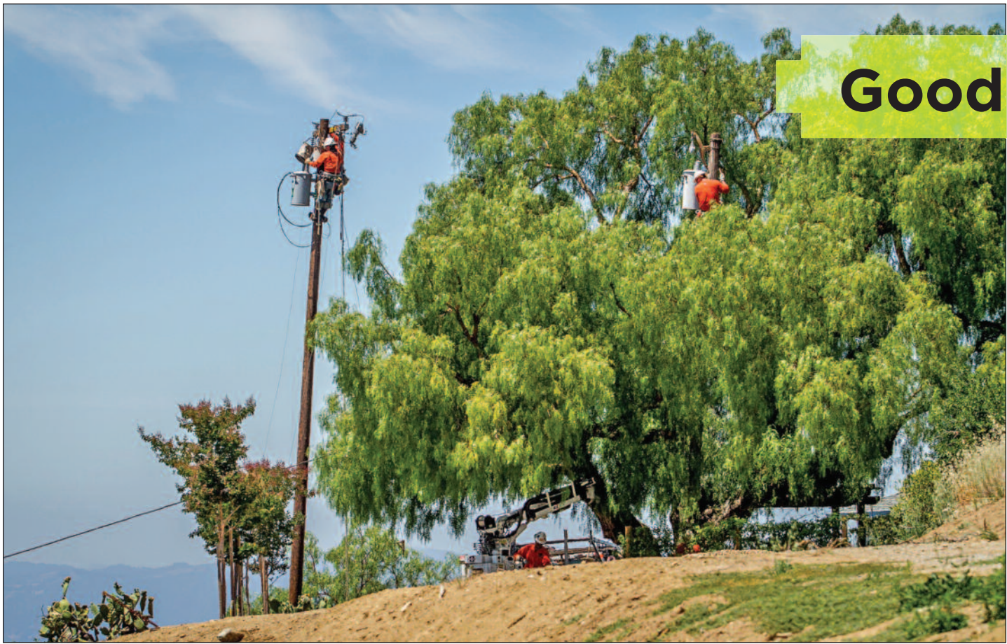
Crew works to move the power lines to the new pole.
