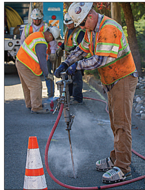
Josh Wisdom uses a pipe locator to find the main, then drills test holes.
