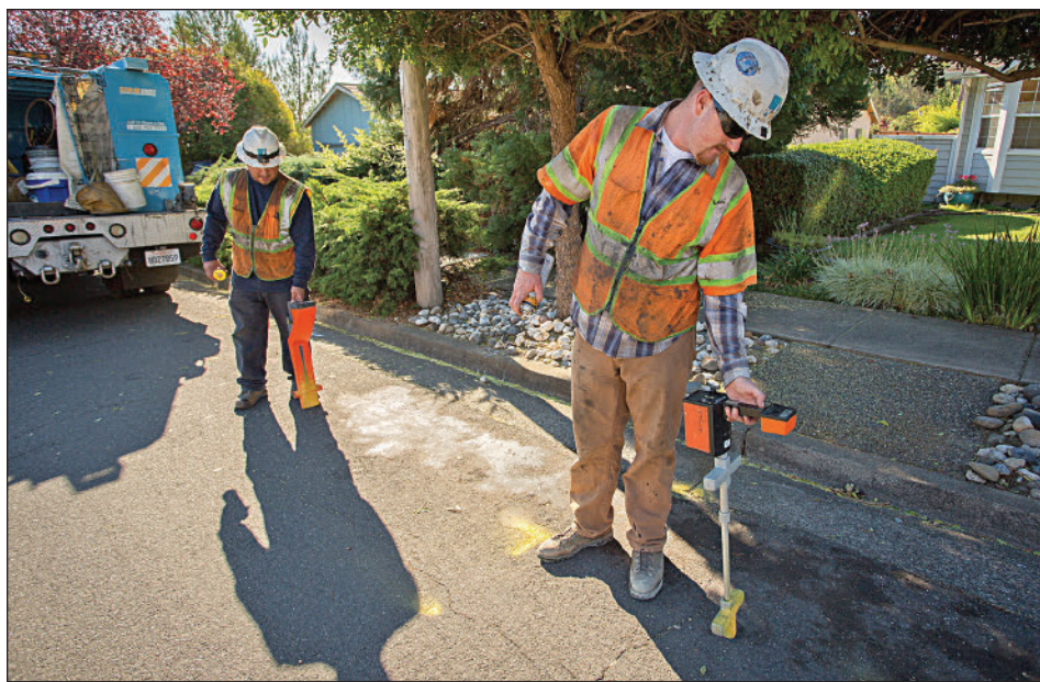
Josh Wisdom uses a pipe locator to find the main, then drills test holes.
