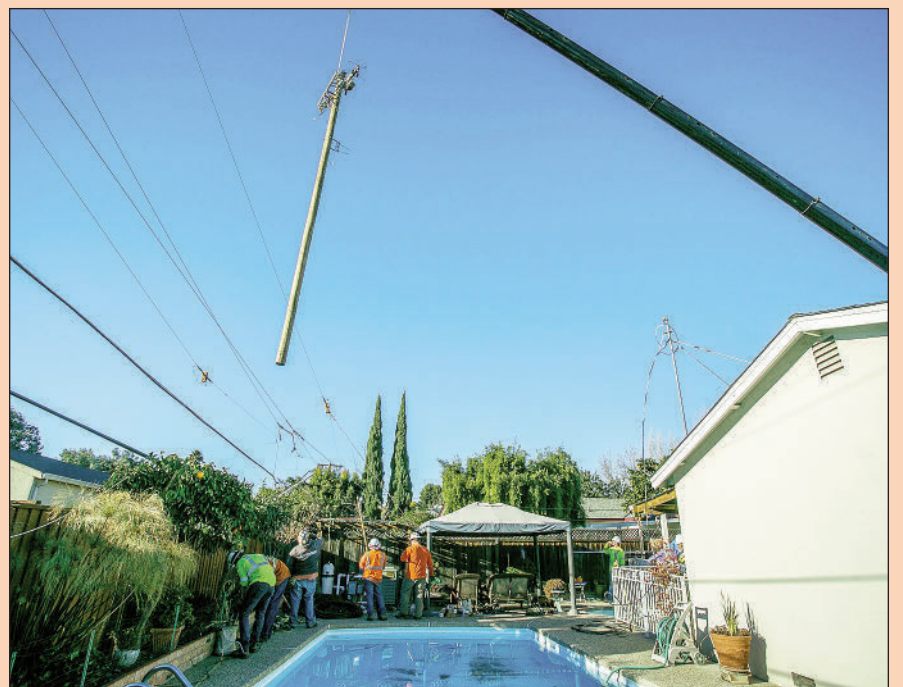
Beginning its descent, the pole will be set in the same hole as the pole being replaced.
