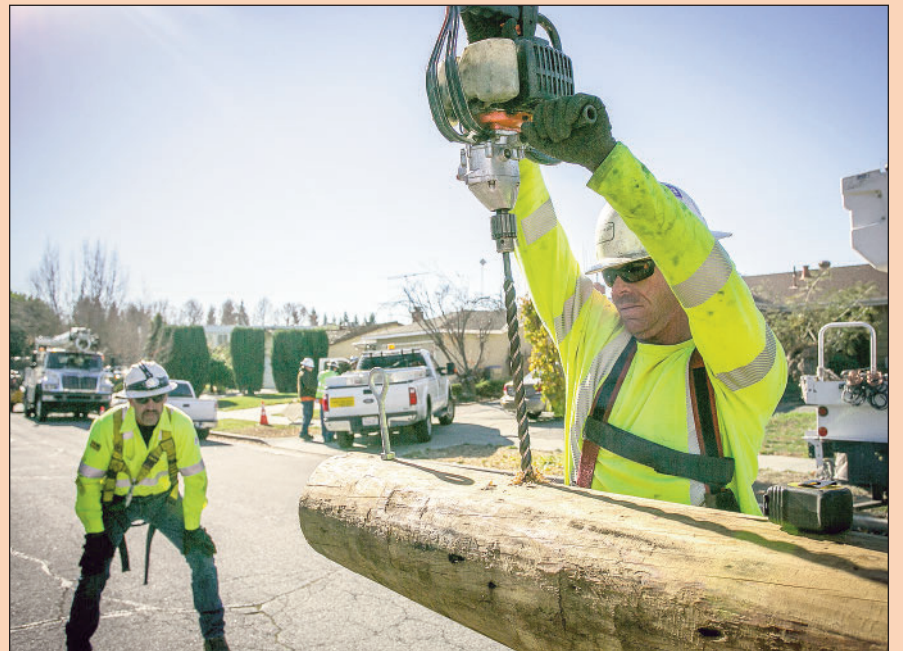
Todd Bryant checks the angle while Matt Petesch drills into a new pole that will be lifted over a house by crane. Both IBEW members are journeyman linemen for Henkels-McCoy. Other members working the job were Paul Perrerr, Josh Reneson, Todd Bryant, Jay Karpinski, Seth Rall, Nick Jonson, John Llorca, Hiram Vidal, Steve Murillo, Jonathan Barragan and Chris Mendoza.
