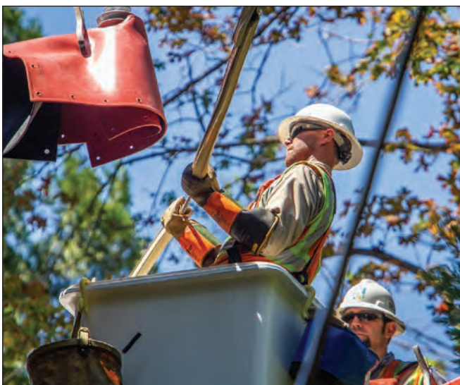
[ABOVE AND RIGHT] Anthony Albright, left, and Adam Beene install rubber.
