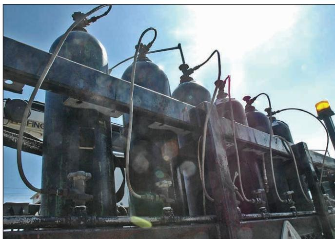
[LEFT] Nitrogen is used to blow the "pig" to the pulling end of the job, where it is attached to a cable line, which is dragged back to the end where the cable spools are located. The cable line is then attached to a "head" where all three cables come together.
