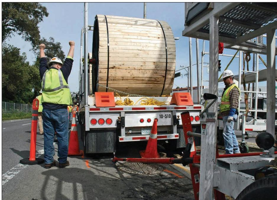
Stop right there! The cable spools have to be aligned just right. A bad angle at the front end of the pull would be amplified en route to the other end—causing the cable to bind up.
