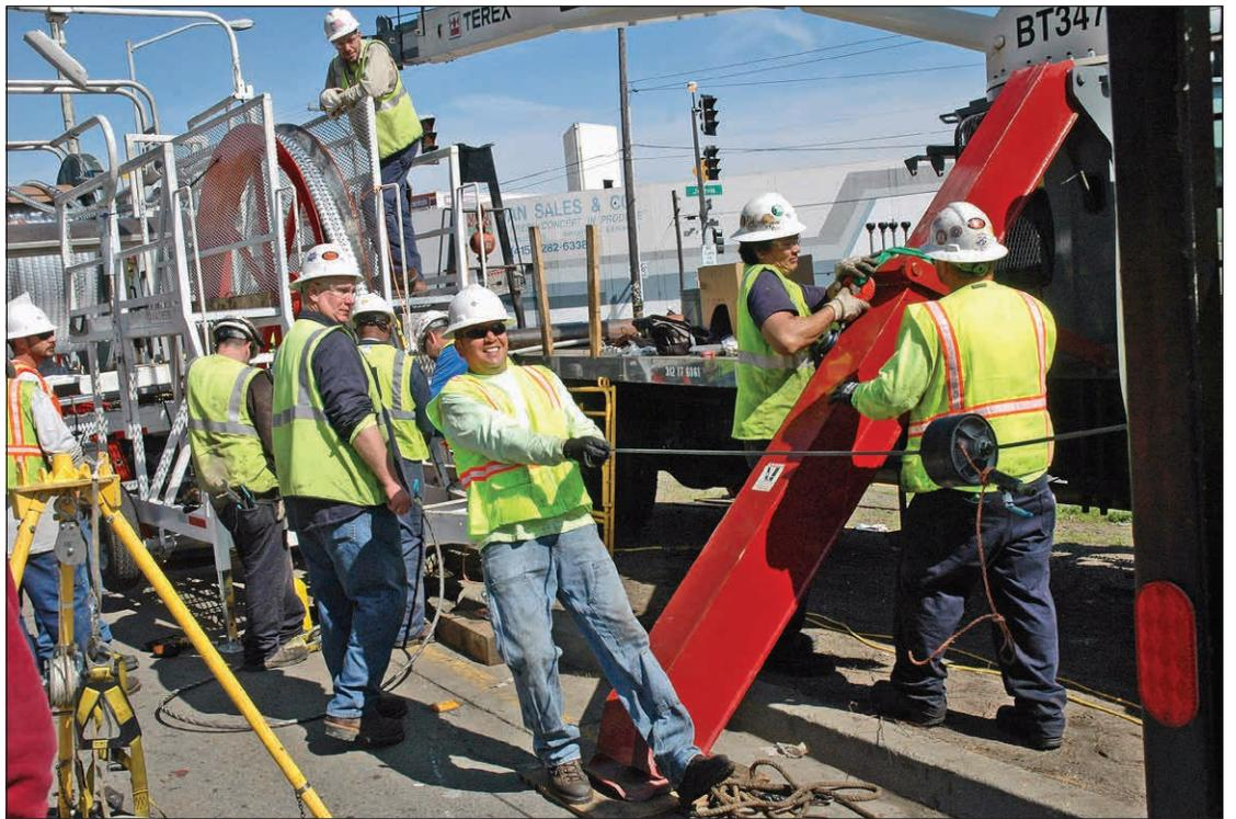
[ABOVE] Just got the hardline in; now reeling cable up on the nitrogen truck to get it out of the way.
