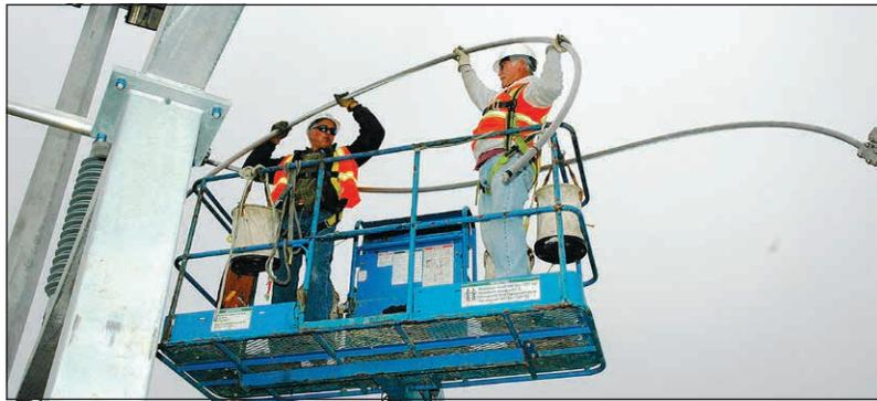
Evans and Trillo installing jumpers to 115 kv breaker.
