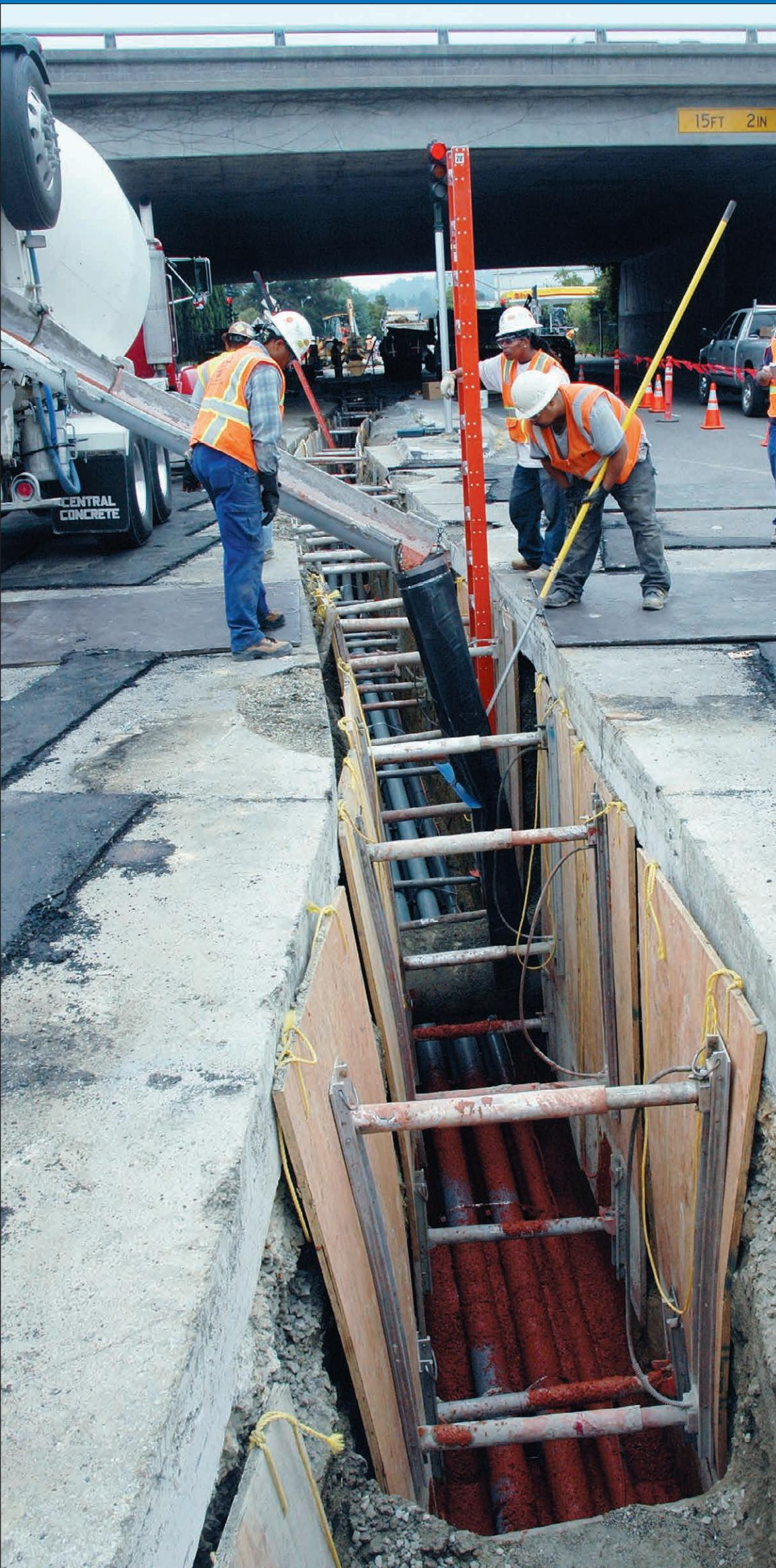
The trench is shored and the conduit laid as the job progresses up Park Blvd. in Oakland. In the distance, the excavator extends the trench under Interstate 580. Pouring a specially designed thermal cement that will help dissipate heat generated by the electricity in the cable are, from left, Technicians Daniel Wheeler, Tonisha Tizeno, and Douglas Castillo (bending down).
