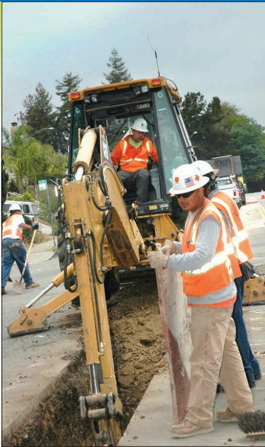
Equipment Man Del Schellenger digs the trench with the excavator. Technician Rosendo Herrera stands ready with the shoring.
