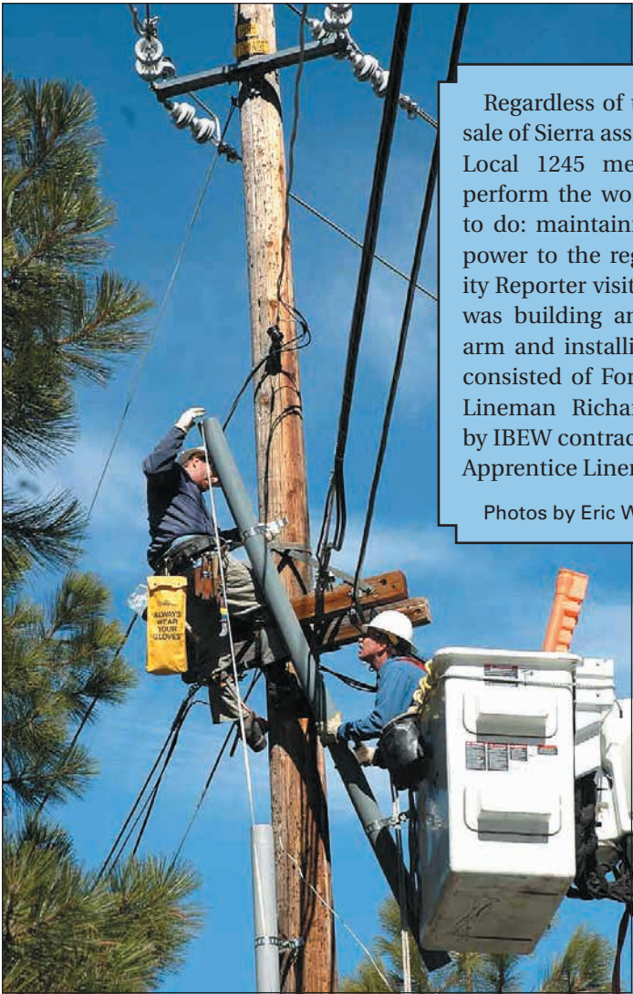
Dillard and Tracy maneuver the top segment of the riser into position.
