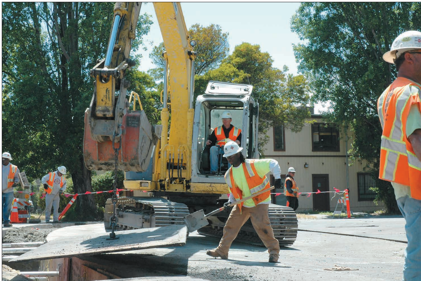
The trench has to be covered back up at the end of each workday.
