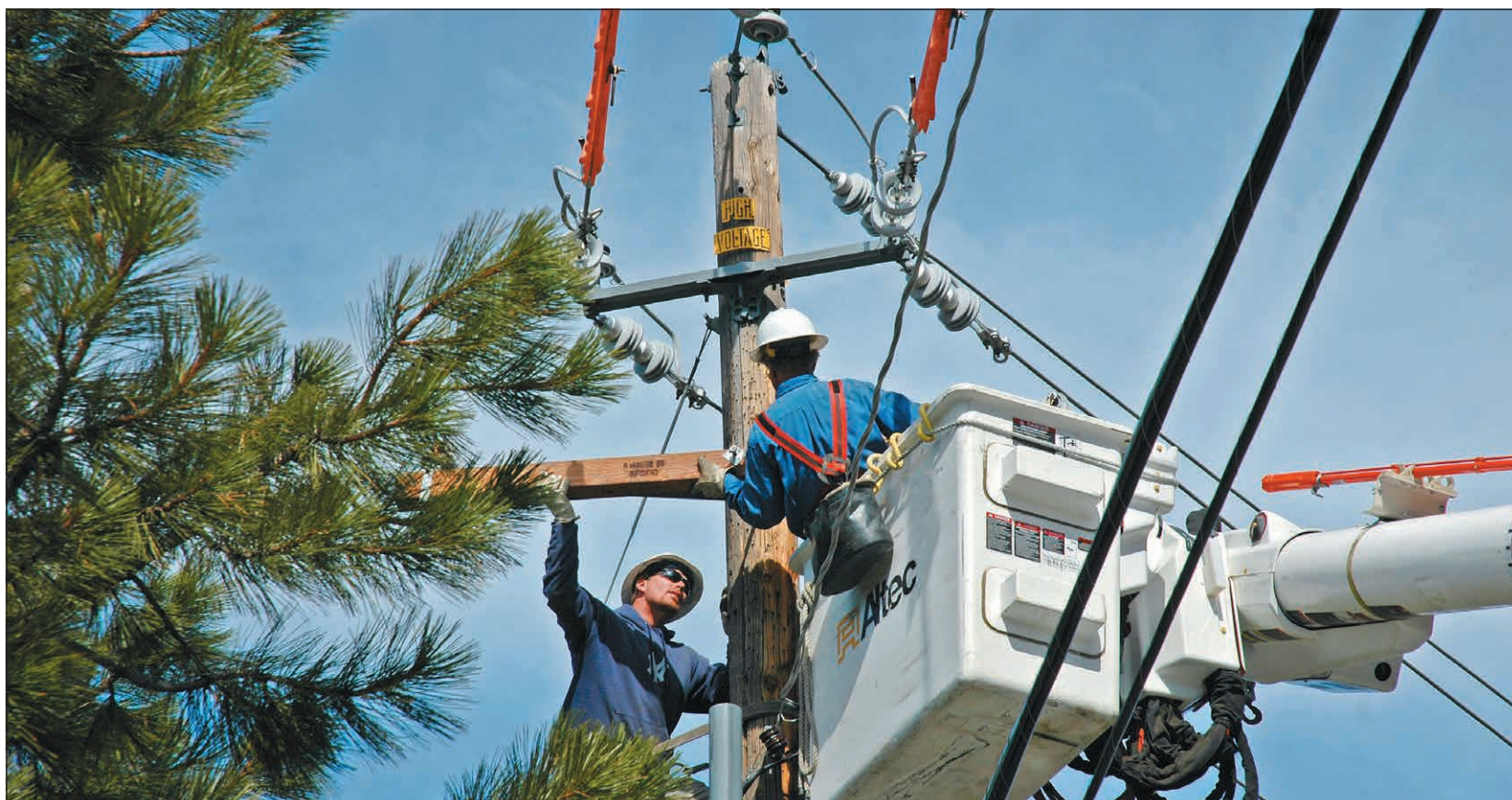
Jared Dillard, on the pole, and Richard Tracy, in the bucket, maneuver the new crossarm into place.
