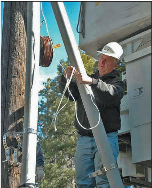
Steve Bottrell preparing the riser for installation.
