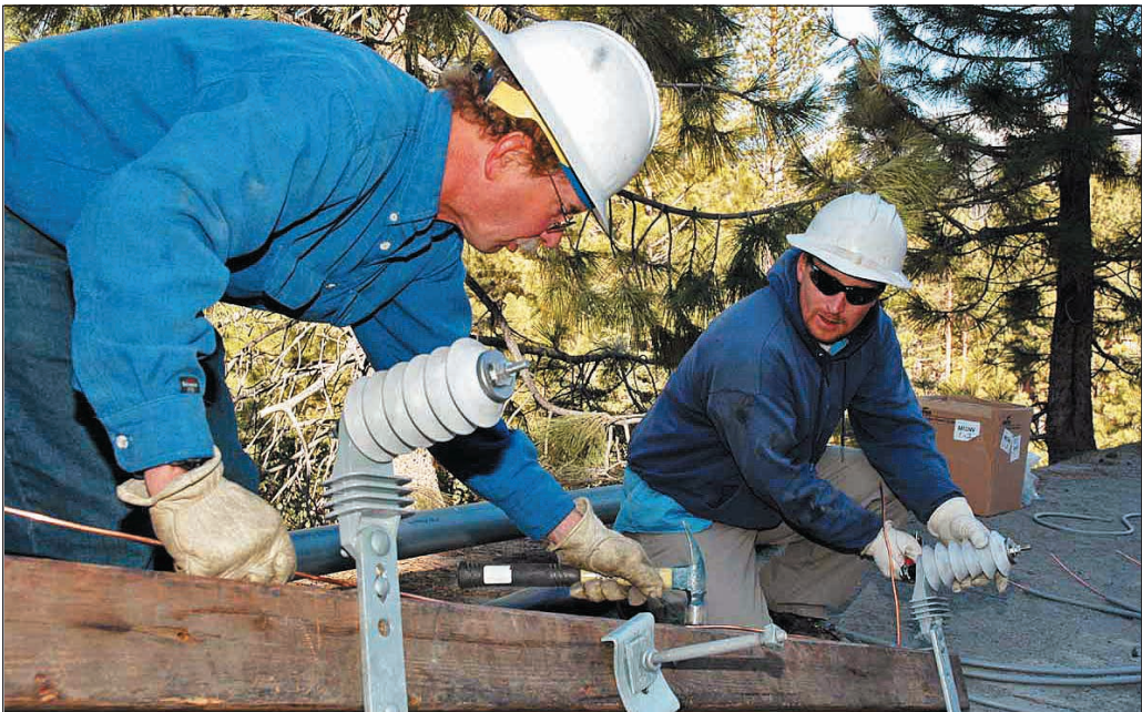
Richard Tracy, left, and Jared Dillard build the new crossarm on the ground.
