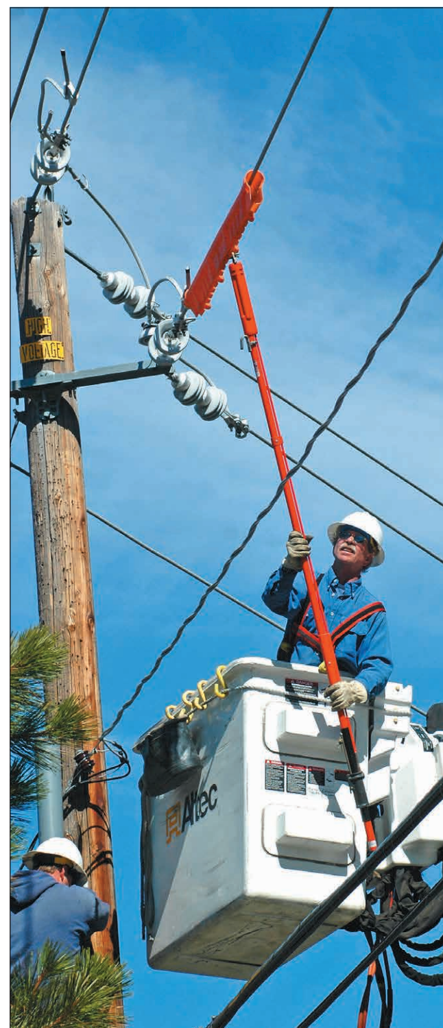
Richard Tracy cover an energized line with the orange snake.
