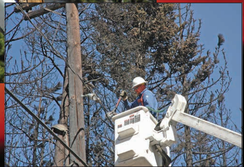
Paul Deusing, Sierra Pacific Power Troubleman out of Reno, hangs secondary on Mt. Rainier Drive.
