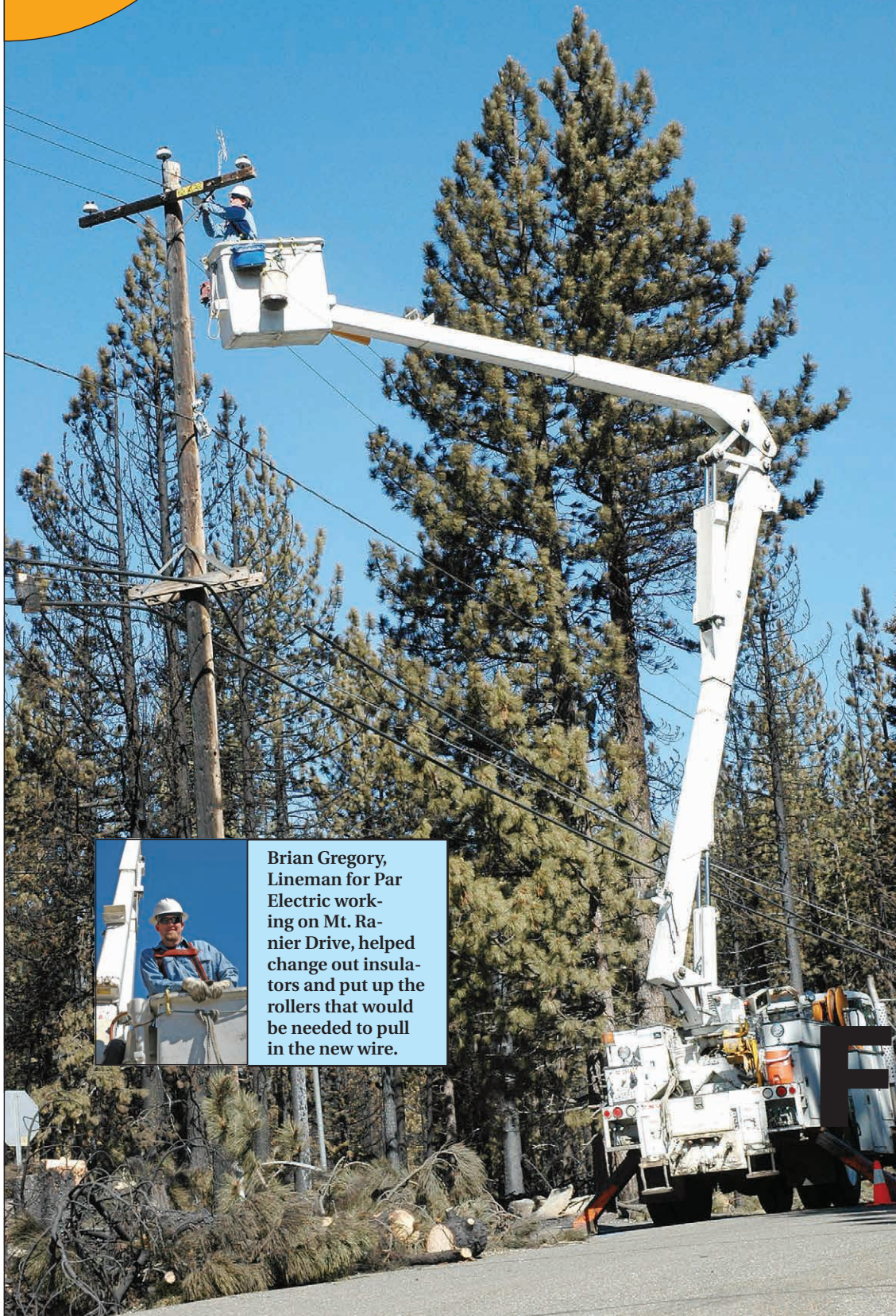
ABOVE RIGHT: Par Electric Lineman Ross Phillips changes out burnt glass for new glass, prior to hanging rollers for stringing new wire. "We were rebuilding the main feeder for that area so the people who had houses left could have power ASAP," Phillips said.
