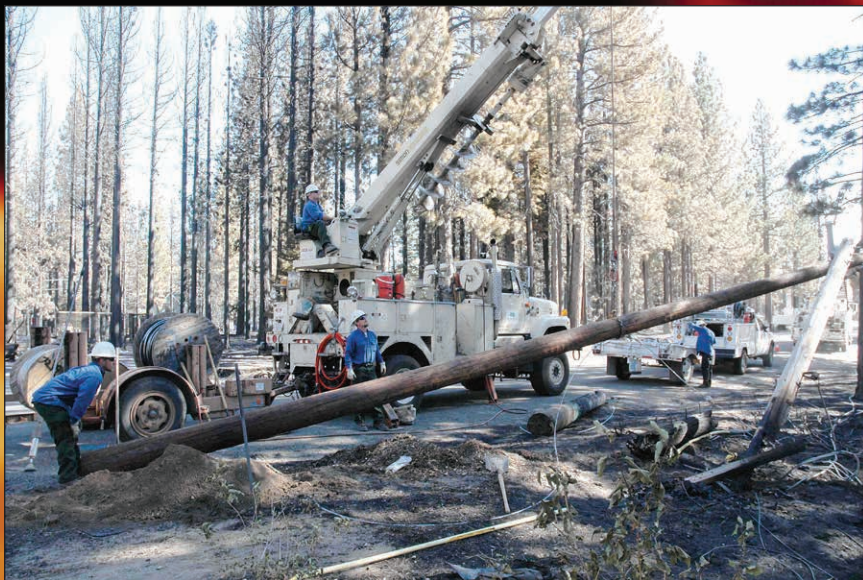
Local 1245 crew sets a new pole to replace one destroyed by the fire. From left are Apprentice Lineman Jon McCue, Foreman Garrett Smith, Lineman Justin Wearin (operating bore), and Lineman Marc Christensen.
