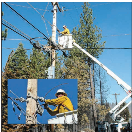
Sierra Pacific Power Troublemans Brian Valencourt hangs secondary wire on Mt. Rainier Drive in South Lake Tahoe.
