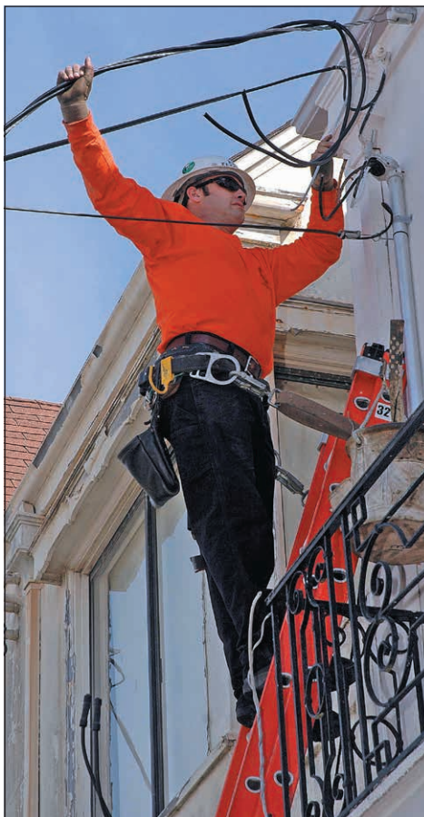
Jason Clause attaching new service to a house and making the weatherhead connections.
