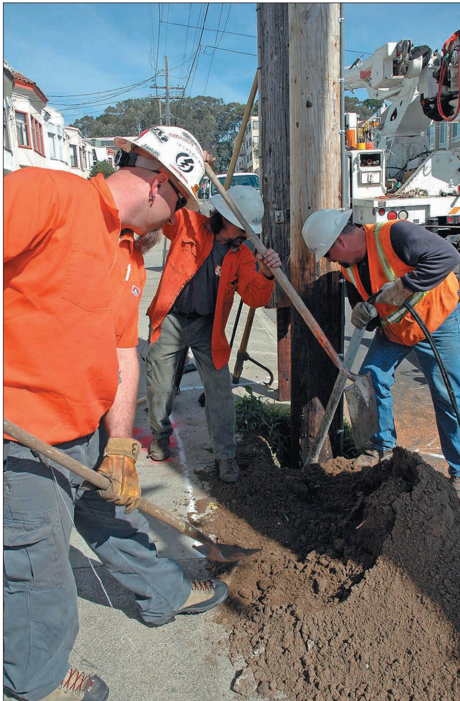
Packing fill around the base of the pole are, from left: Casey Kelly and Marshall Free, shoveling dirt, and Donald Mathews running hydraulic tap.
