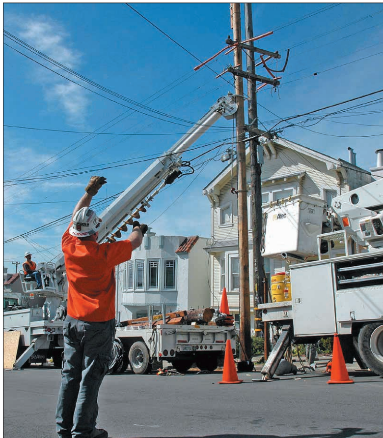
Casey Kelly uses a plumb line to make sure the new pole is level.
