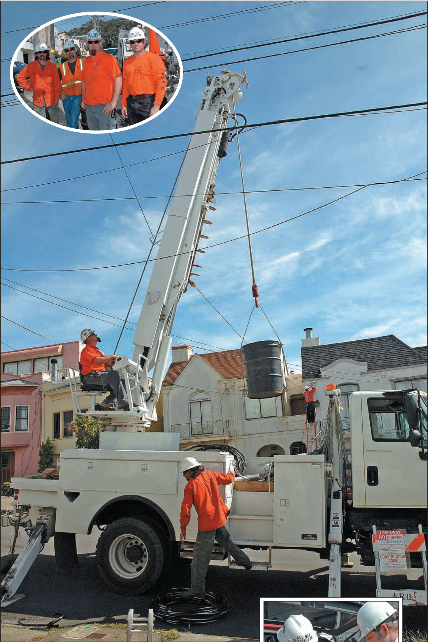
Casey Kelly picks up a bucket of fill to pack around the newly-set pole.
