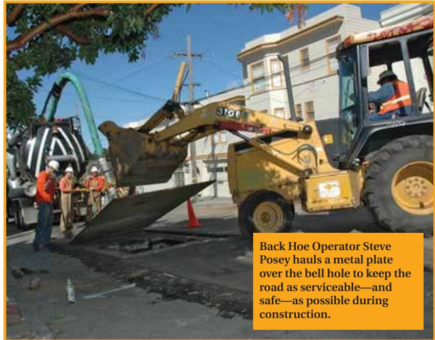
Back Hoe Operator Steve Posey hauls a metal plate over the bell hole to keep the road as serviceable—and safe—as possible during construction.
