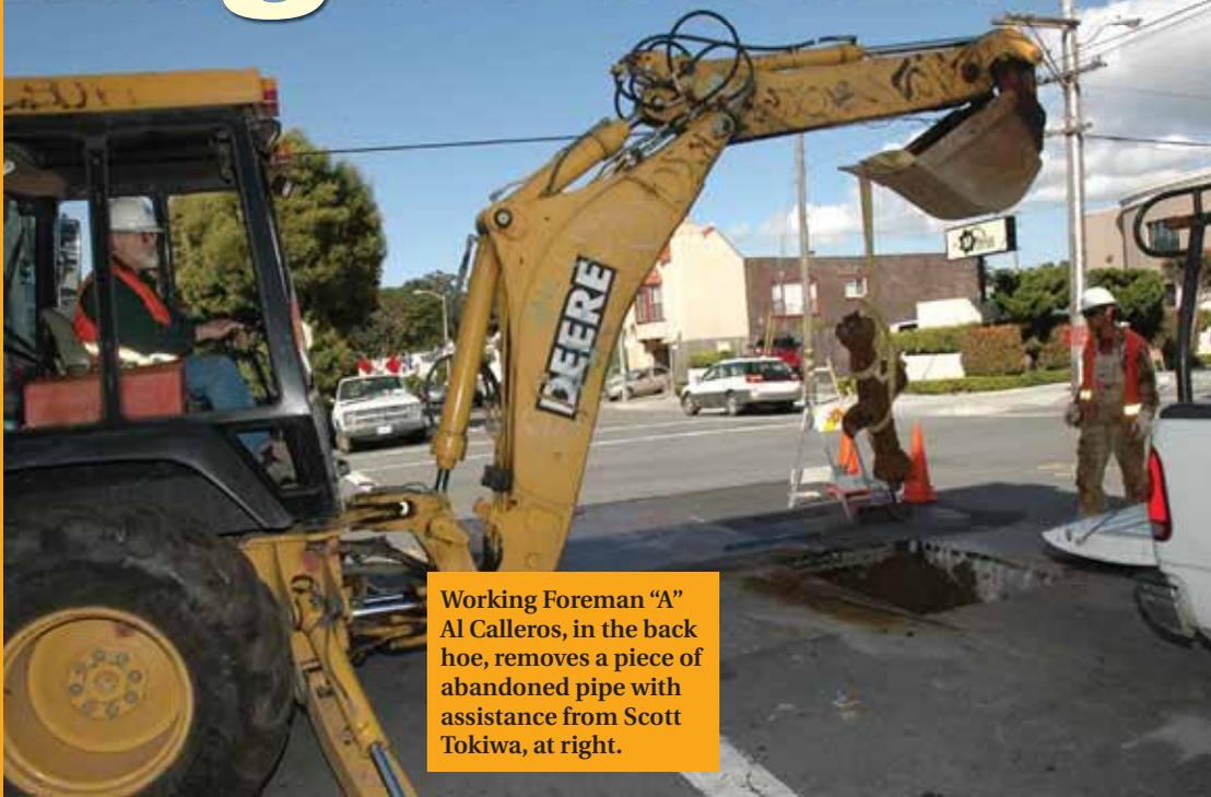
Working Foreman "A" Al Calleros, in the back hoe, removes a piece of abandoned pipe with assistance from Scott Tokiwa, at right.
