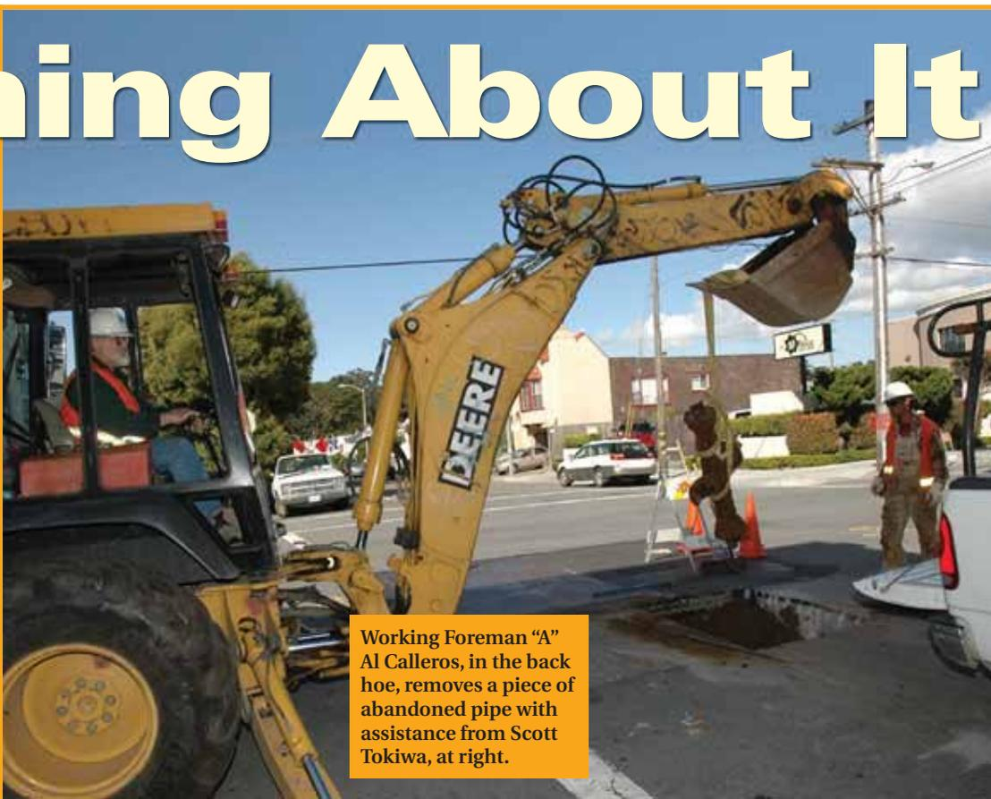
Working Foreman "A" Al Calleros, in the back hoe, removes a piece of abandoned pipe with assistance from Scott Tokiwa, at right.
