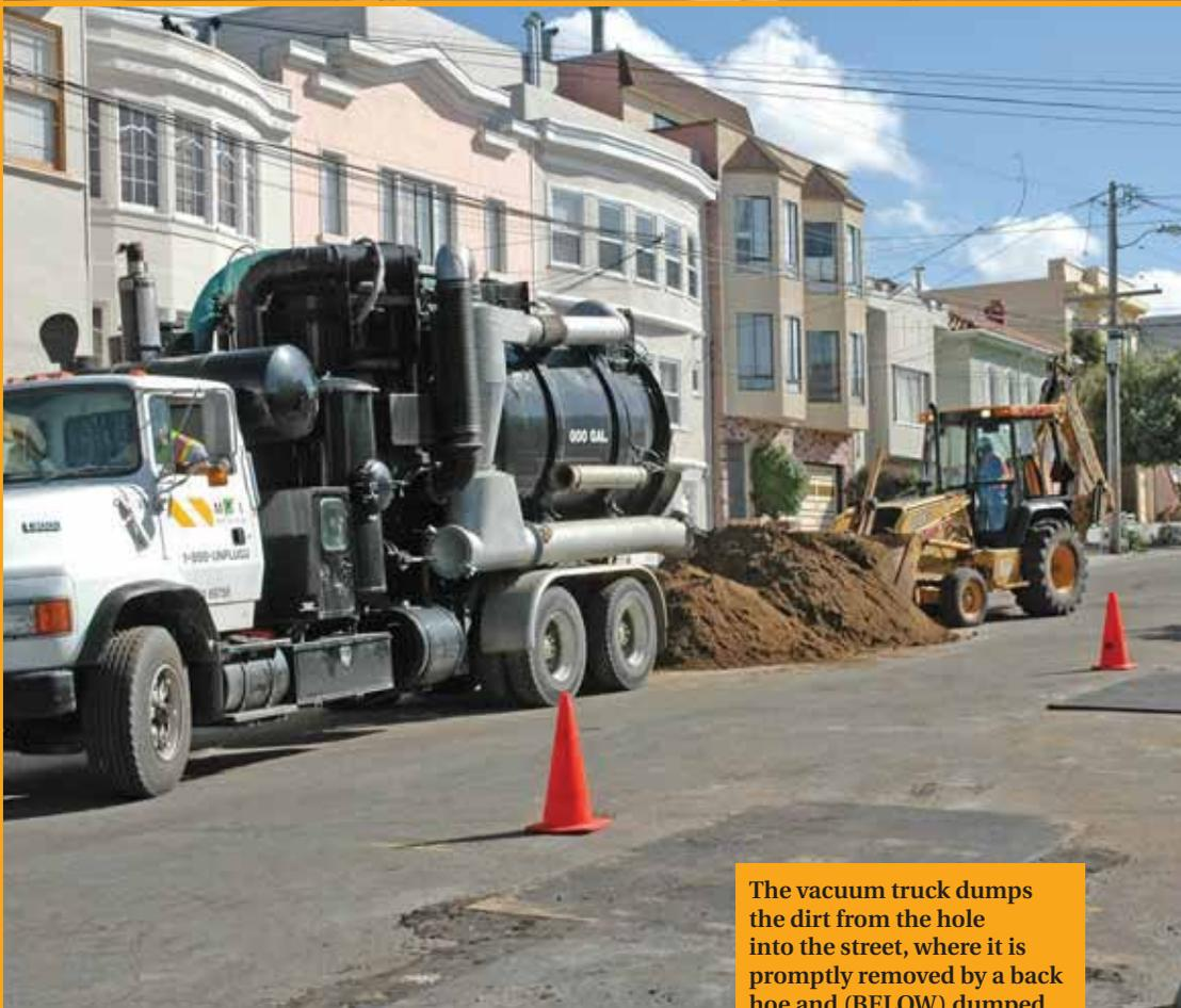
The vacuum truck dumps the dirt from the hole into the street, where it is promptly removed by a back hoe and (BELOW) dumped into a truck for removal.
