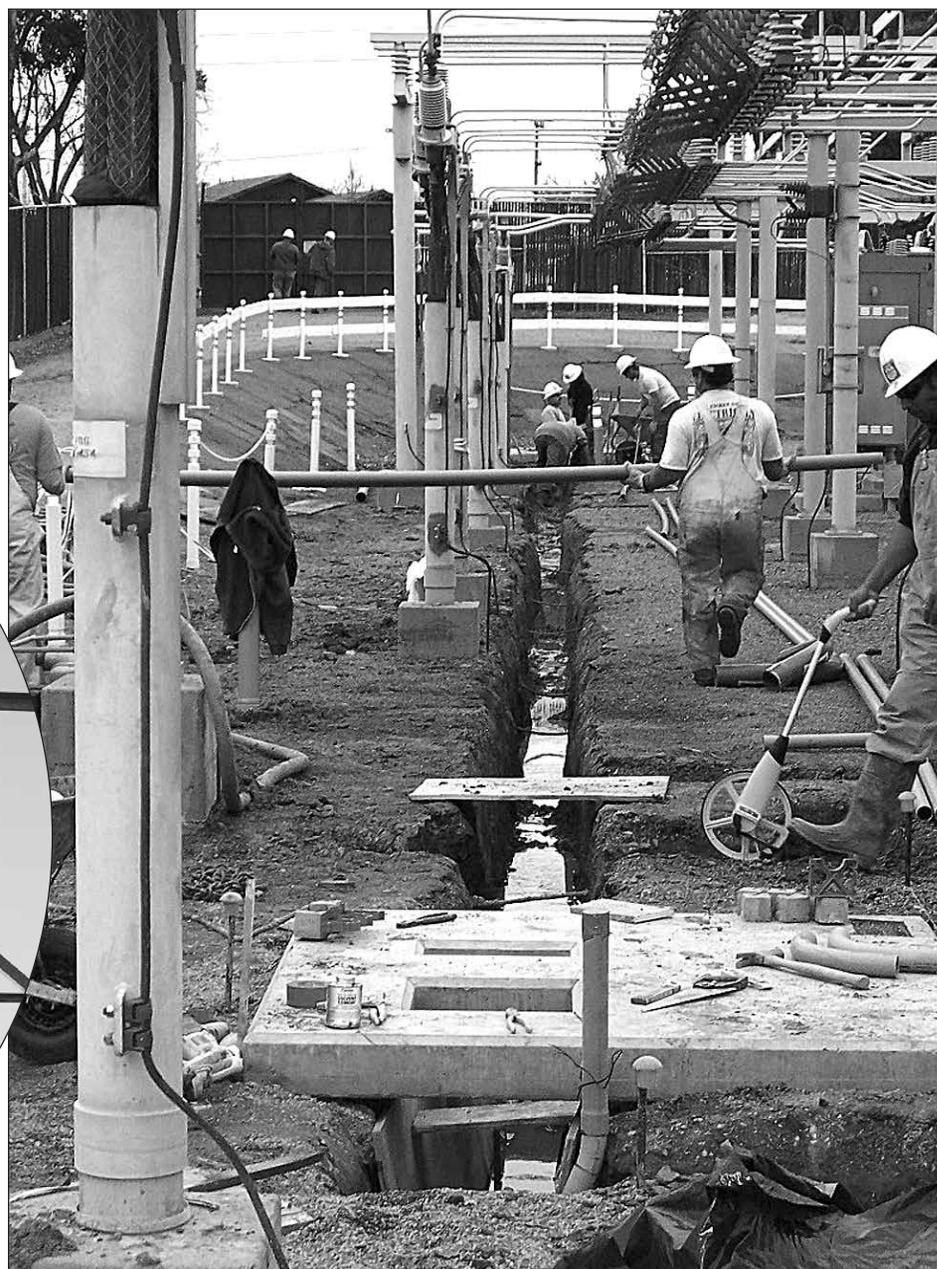
Work in the Vacaville substation installing DCSI electric powerline communications equipment.
