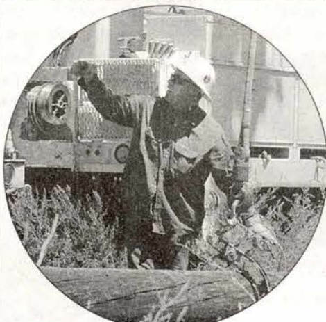
Foreman Jim Seevers disconnects the yacht braid, releasing the stub.
