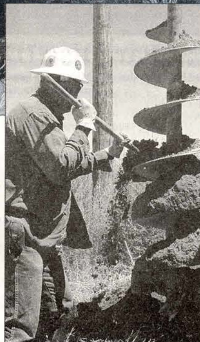
Lineman Bob Helton clears the auger that is drilling a hole for the new pole.
