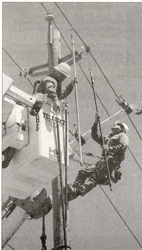
Foreman Jim Seevers disconnects the yacht braid, releasing the stub.
