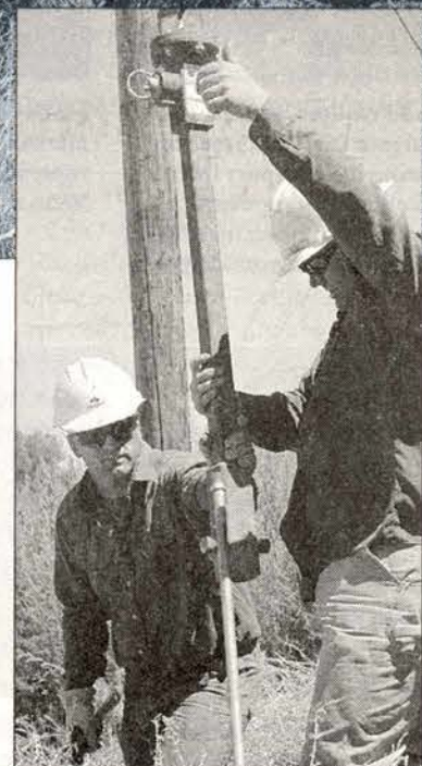
Linemen Reto Gross (left) and Bob Helton install the screw anchor.
