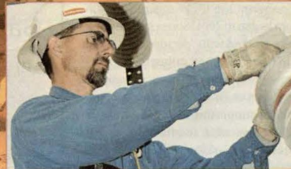
Greg Lloyd, Substation Electrician, hooks up jumpers at the new Kiernan Substation.
