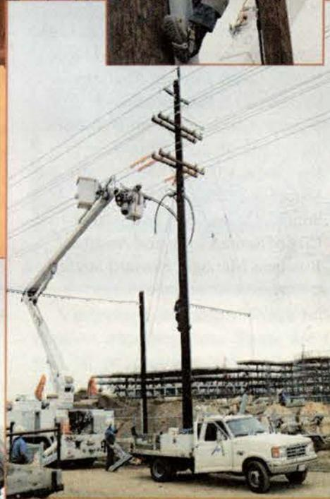
ABOVE: MID crew pulls in underground wire for a new Kaiser facility (under construction in the background).
