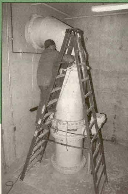
John Woods, Mechanic, working on influent valve to floculation basin.
