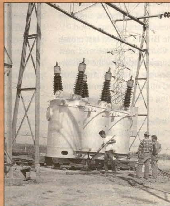
Ready to roll out a retired 100 KV OCB at Semi-Tropic Substation are Jerry Wells, Relas Powell, and Rodger Hughes.
