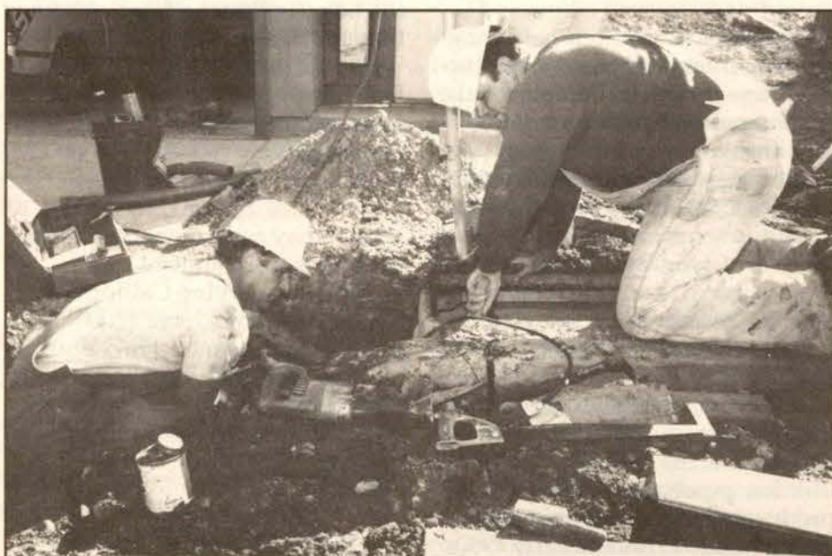
Gas Crew Foreman Andy Dakopolos (left) and Utility Worker John Tiemeyer, both Local 1245 members at PG&E, install half-inch gas line and electric conduit to newly-rebuilt residences in Hiller Highlands, an area ravaged by the 1991 East Bay fire. (Photo: Eric Wolfe)
