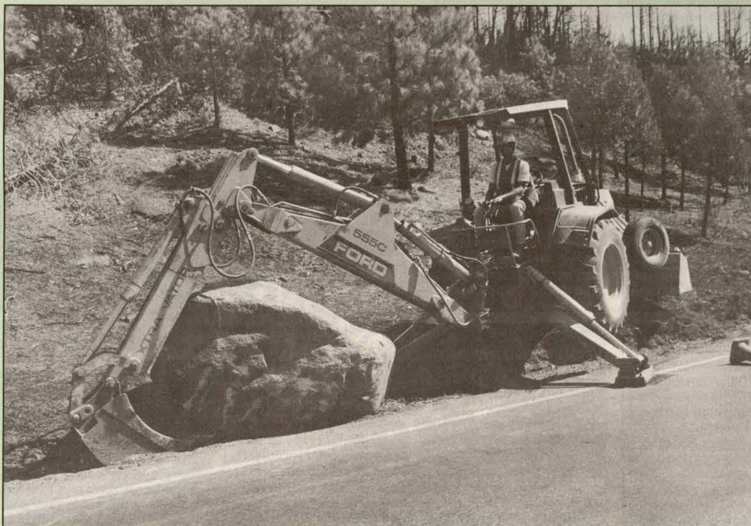
Large boulders provided the chief obstacle to laying new underground cable. (Photo: Tony Gomez)
