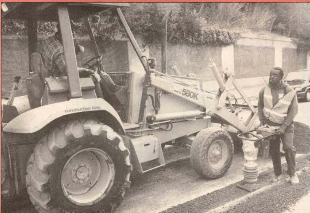
Gas crew foreman and 22-year union member Will Warren operates the whacker on Broadway gas main construction job.
