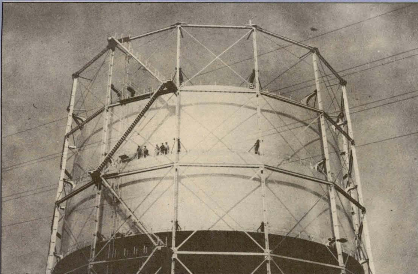
Crew greasing lifts on low pressure water lift gas holder at PG&E's Stockton Gas Plant in 1951. (Courtesy Ken McAuley)
