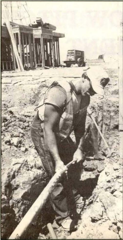
BRINGING GAS TO LAGUNA Darryl Lewis, PG&E gas crew foreman and a 24-year union member, assembles a gas riser (below) as he and Fieldman Bruce Jenkins (above), a six-year union member, install half-inch plastic conduit services in the Laguna Meridian No. 1 development south of Sacramento, Ca.
