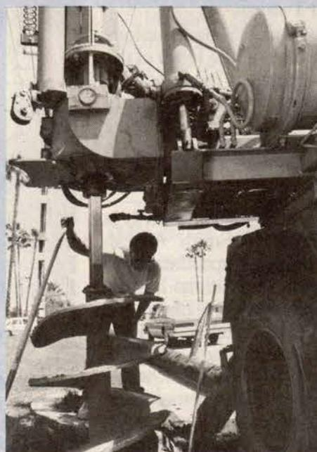
Setting a 90-foot pole in place are (above, from left) Operator John Dykes, Bob Broussard and Billy Reed. At left, Steve Hesse (on the ground) and operator Larry Mascari dig a hole, taking care to not interfere with other services (such as telephone or water) that may be buried in the immediate area. Other union members working for Pouk & Steinle in the immediate area but not pictured are Bob Sandow (steward), Mike McKinney, Ron Pendergrass, and Will Thomas.
