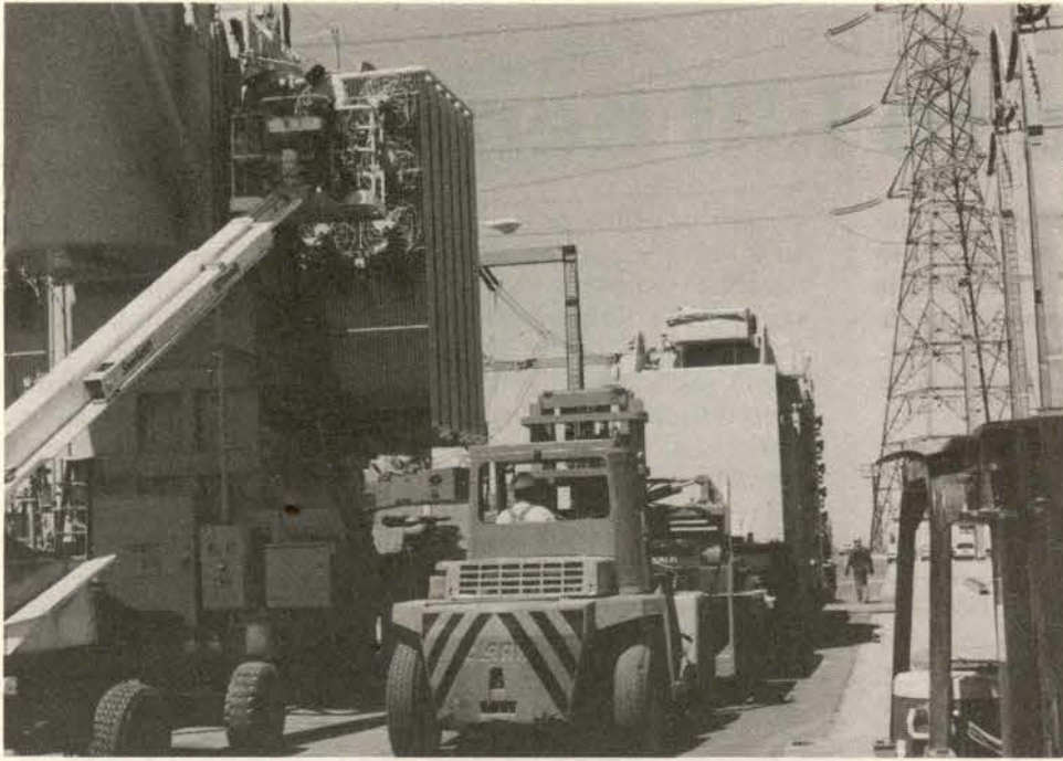
New transformer being pulled in on rail car.
