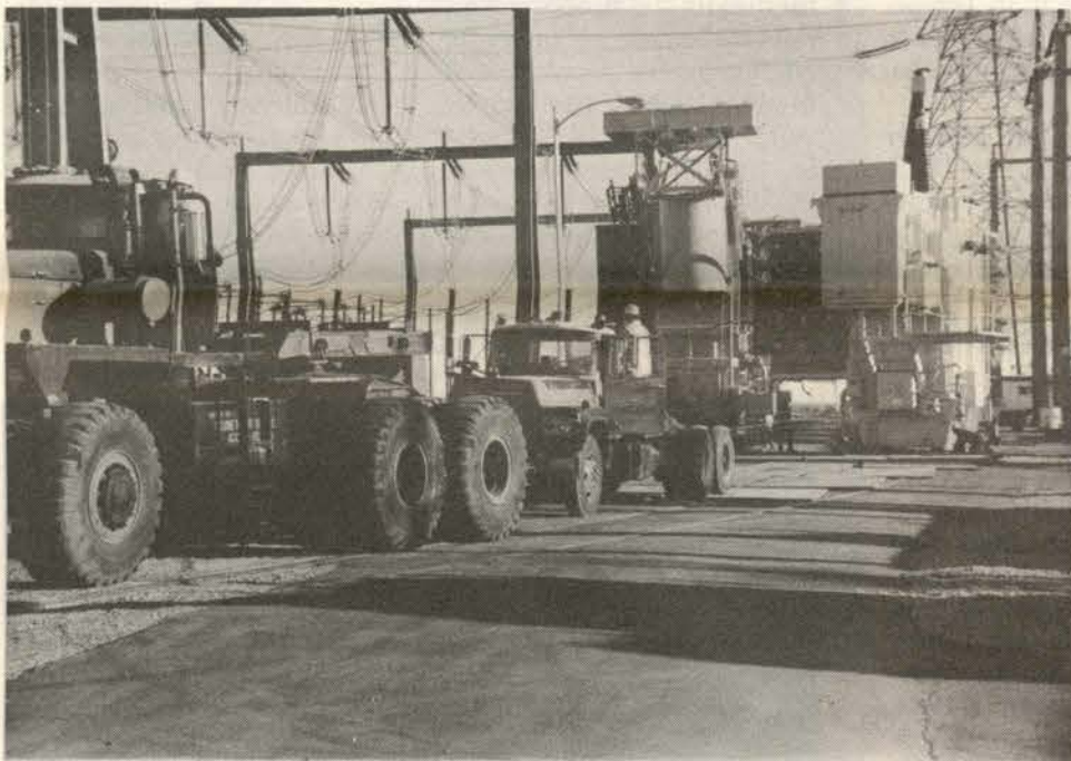
Old transformer and new transformer side by side.
