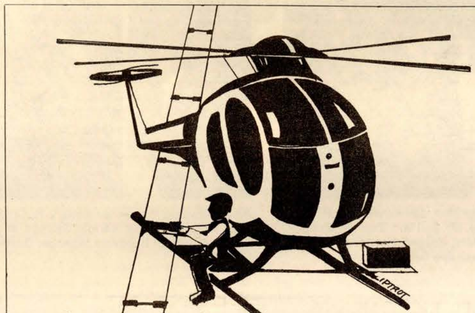
Artist's rendering details worker on helicopter platform adjacent to high voltage line.
