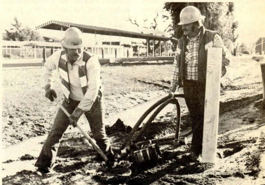
Northeast of Marin County's Ignacio Substation, Sonoma gas crew members are pictured repairing flood damaged lines. Mike Radloff, left, has been with Local 1245 for 12 years, and Glen Poulter, right, is a 22-year Local 1245 member.
