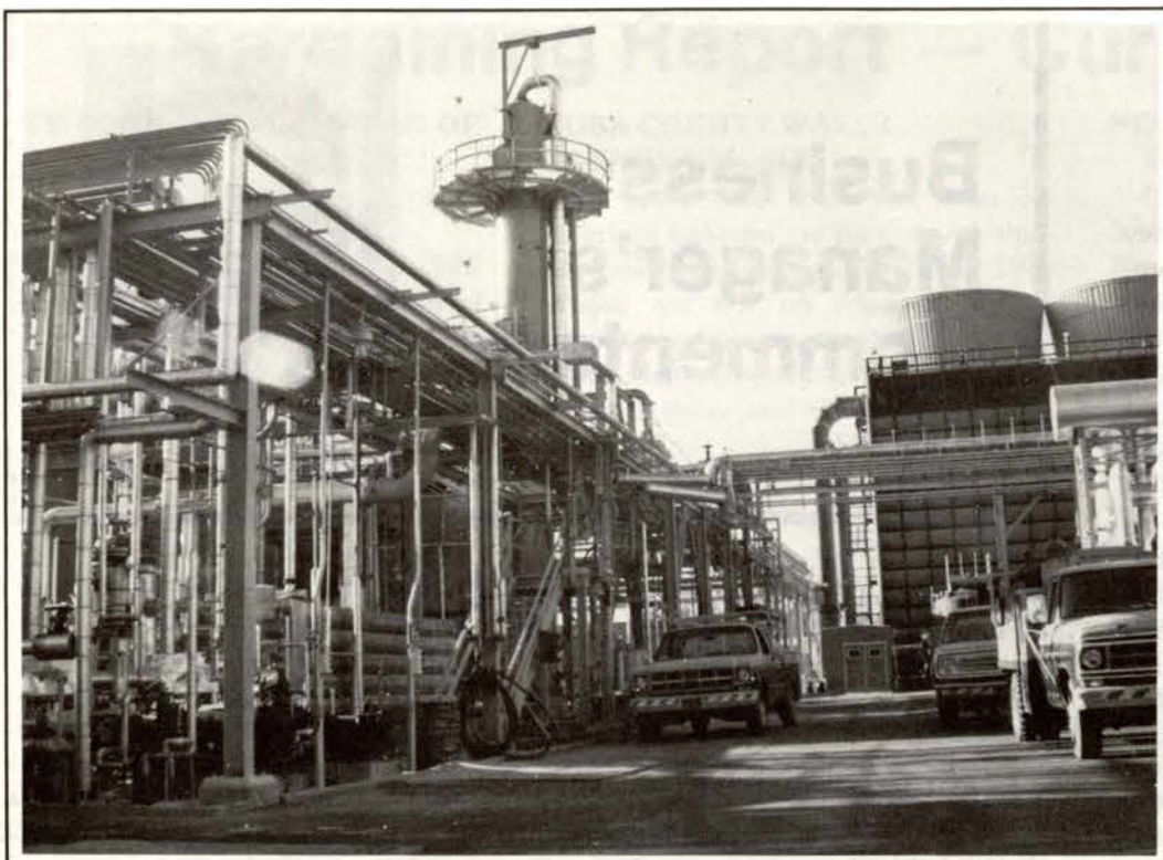
Above: Unit 15's Stretford system was constructed to keep hydrogen sulfide out of the atmosphere.
