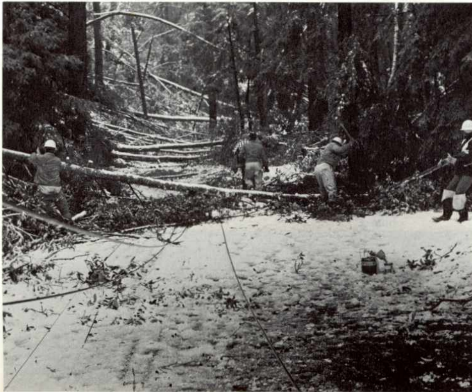
The photo above shows the conditions that our members faced when trying to recover from the January 3rd storm. (The two men without hard hats were evidently local residents helping to clear away brush.) This photo shows Big Basin Way, a main thoroughfare in the Santa Cruz mountains just above Saratoga, Calif.
