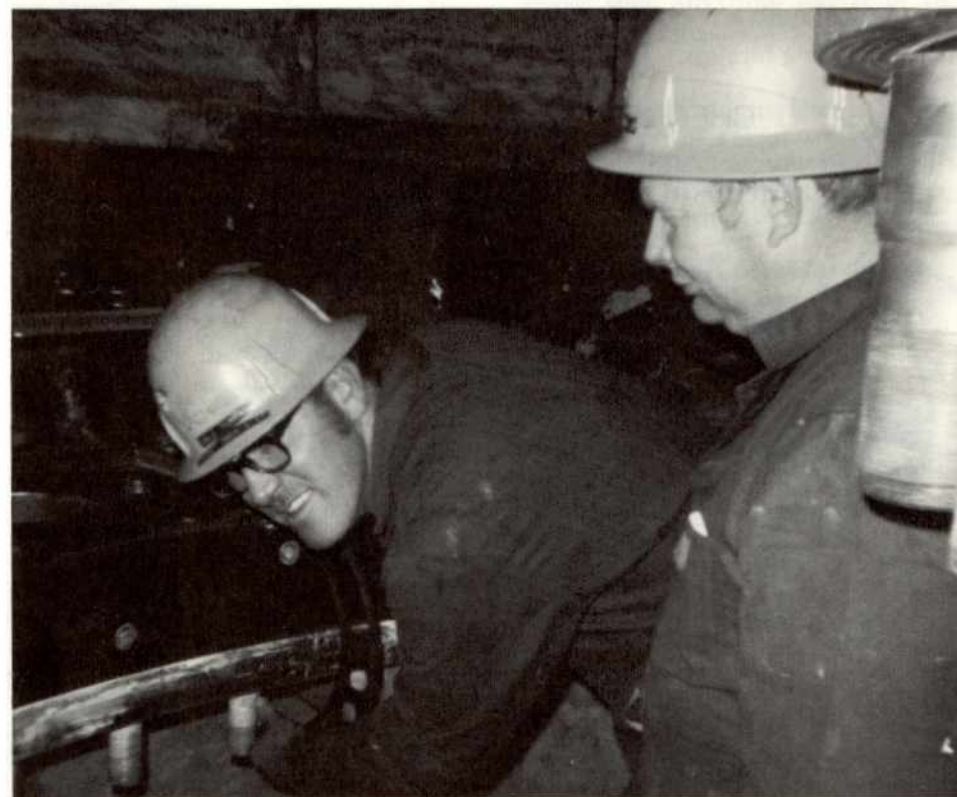
Shown above are Advisory Councilman Dale Turman, left, and Shop Steward Mark Burns taking micrometer readings on lower turbine head.
