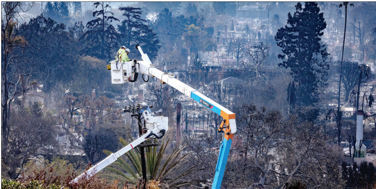
Kern GC Crews doing fire restoration work in Pacific Palisades, CA
