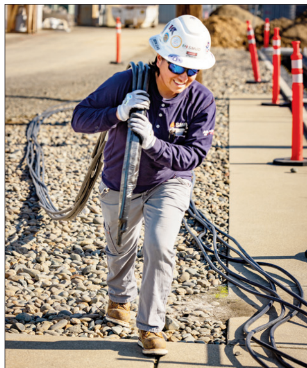
Megan Kilgore, Apprentice High Voltage Substation Electrician
