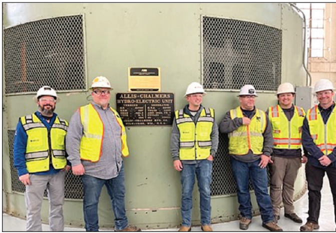
Joseph Klein (SMUD), Brad Early (NV Energy), Pete Winter (SMUD), Johnathon Triplett (PG&E), Aidan McNerney (TMWA) and John Stewart (TMWA) standing in front of unit one at Pit #1 power house north of Burney, CA
