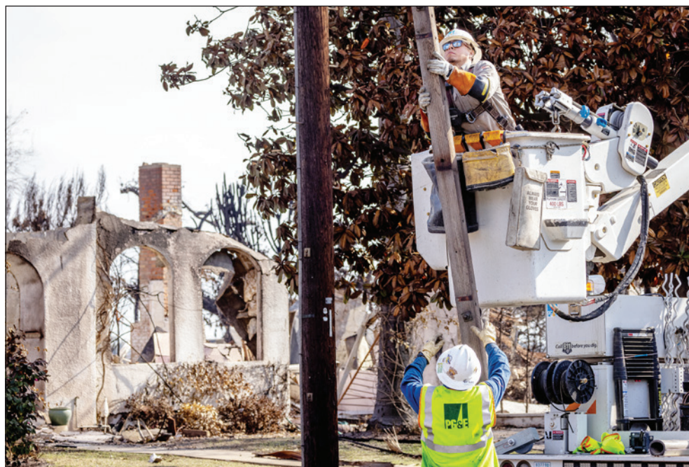
Kern Crews do fire restoration in Pacific Palisades, CA.
