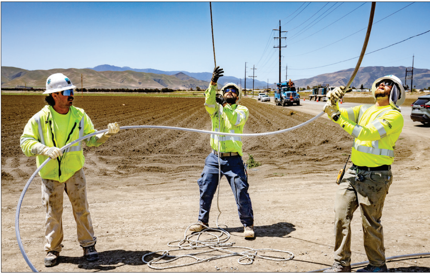
PG&E GC crews on a wire pull in Greenfield, California
