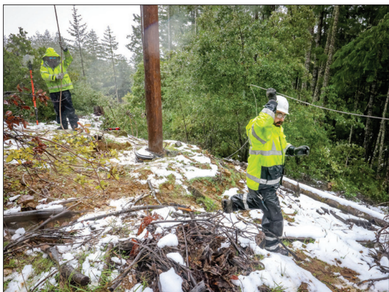
Foreman Kevin Rust, (right), and Lineman Justin McElroy
