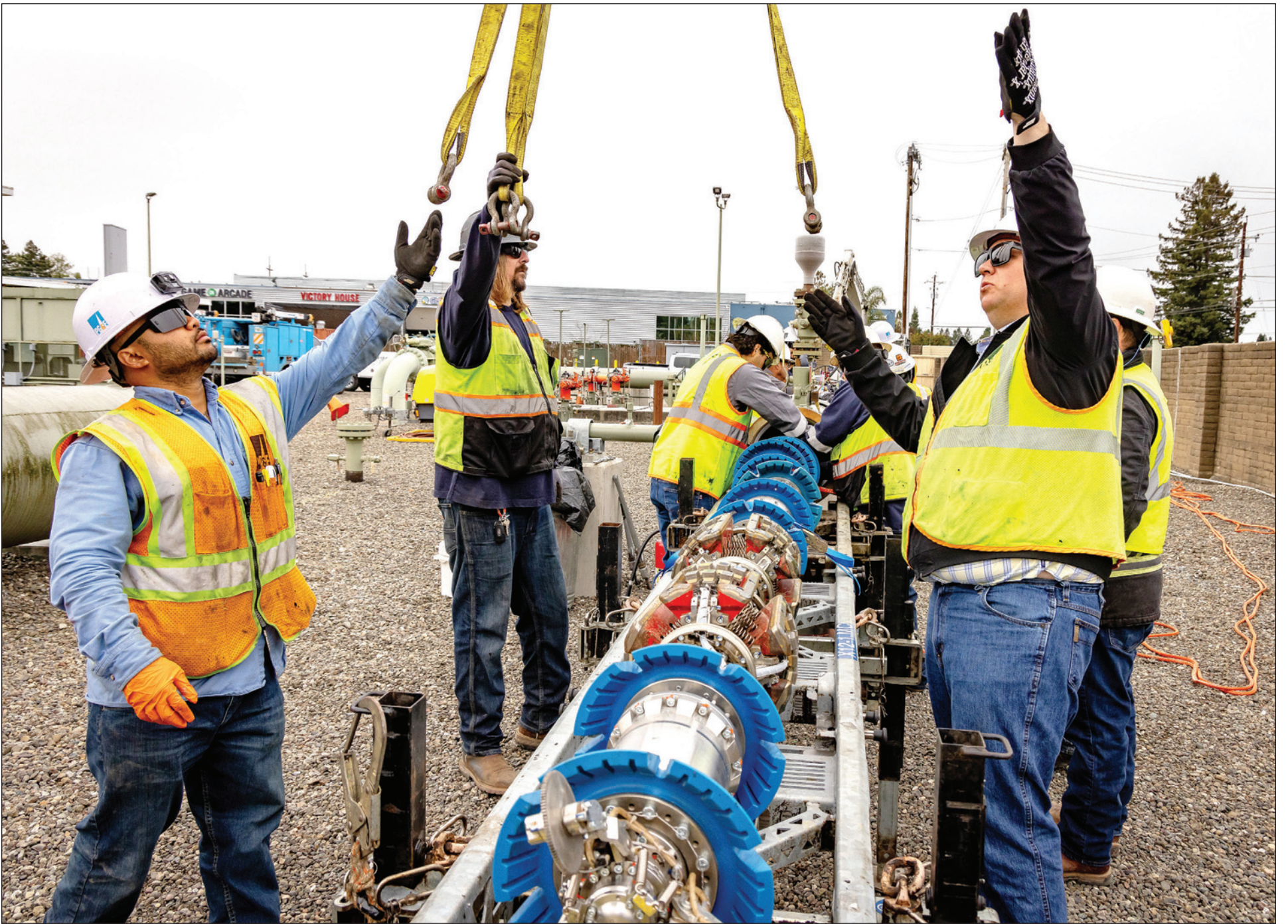
IBEW Local 1245 members from PG&E Gas Department insert a MFLAC tool into the gas main running to Willits from Santa Rosa to check for pipeline anomalies.
