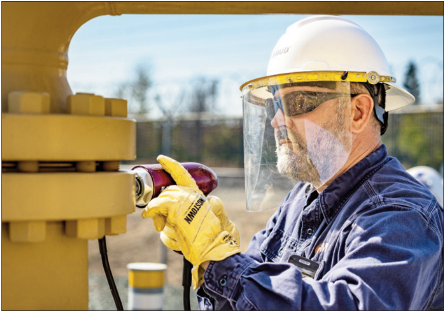
Gas Control Tech George Ordonez performs pin brazing on a valve.
