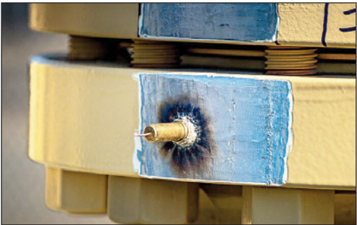
The pin after being brazed onto the valve
