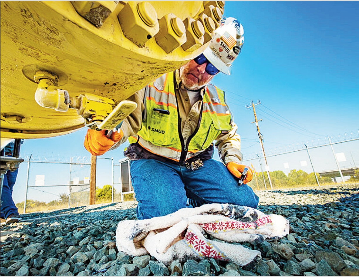
Gas Field Person Jeff Belk tightens a fitting for a valve.
