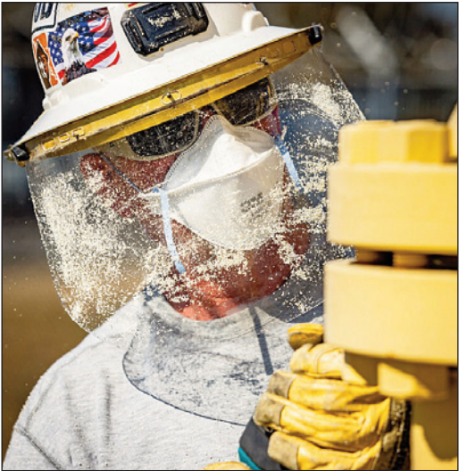
Gas Field Person Rick Anderson sands paint from a valve before pin brazing.
