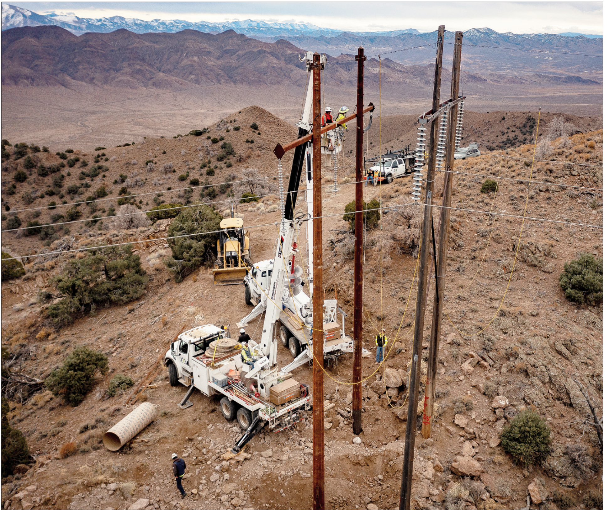
An IBEW 1245 outside line crew from Mountain Engineering worked over the holidays to upgrade a 230KV transmission line located 60 miles from the nearest town of Fallon, NV.
