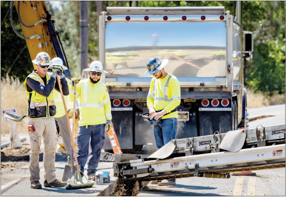
IBEW Local 1245 outside line members working for Dars Cox Construction lay underground conduit for PG&E in Cottonwood, Calif. Photo by John Storey
