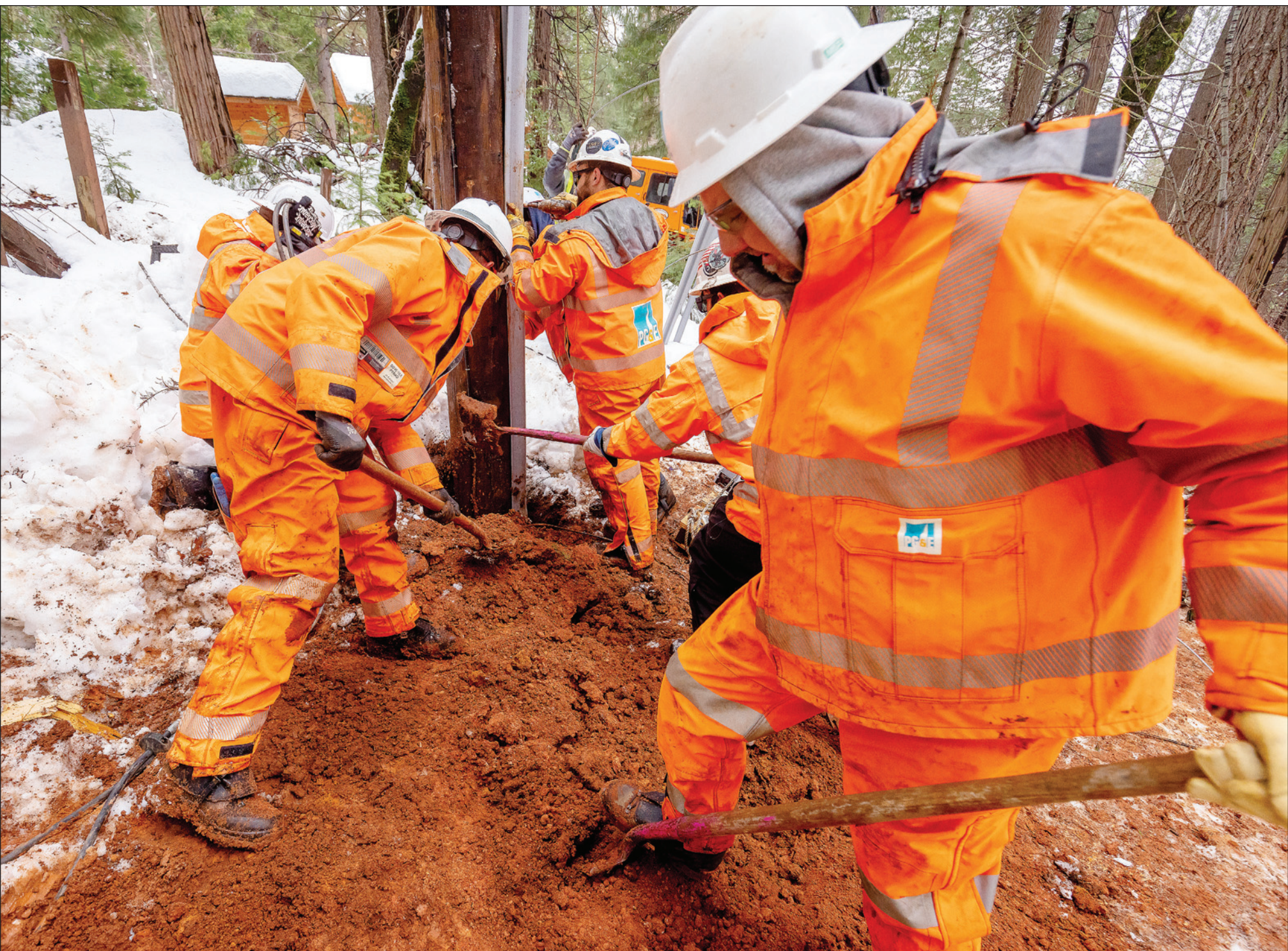
Crews dig and position a pole to restore power on March 9.
