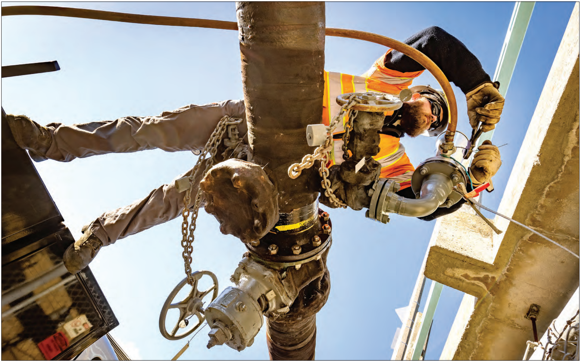
Utility Technician Bradley Bond. Island Energy crews prepare to switch their gas system to CNG so contractors can replace a gas line on the Mare Island Causeway in Vallejo.
