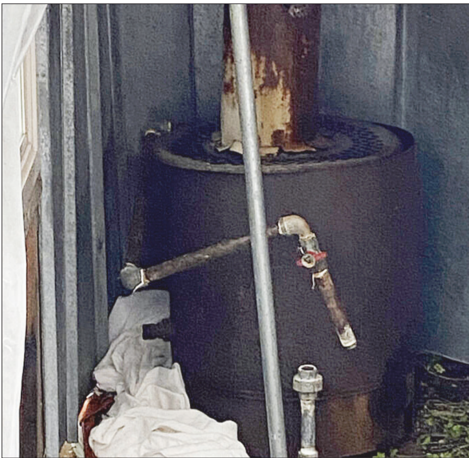
The disconnected gas pipe inside the makeshift sauna.
