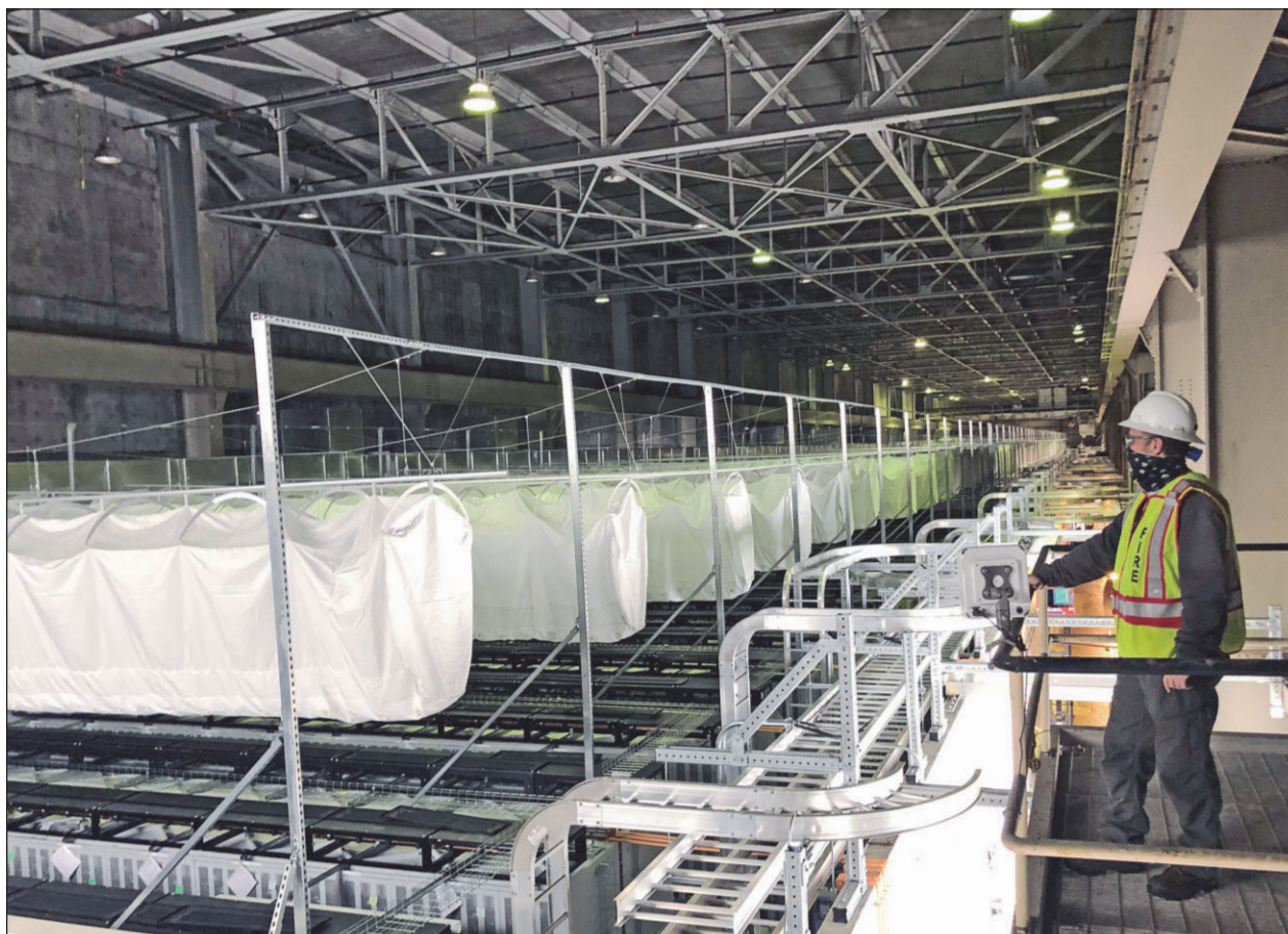
The 300-MW 1,200-MWh battery storage system housed inside the plant's former turbine building
