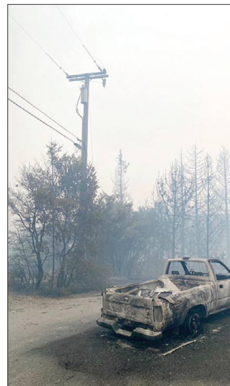
The utility pole in the background was treated with retardant by the SIPT crew, and made it through the fire.
