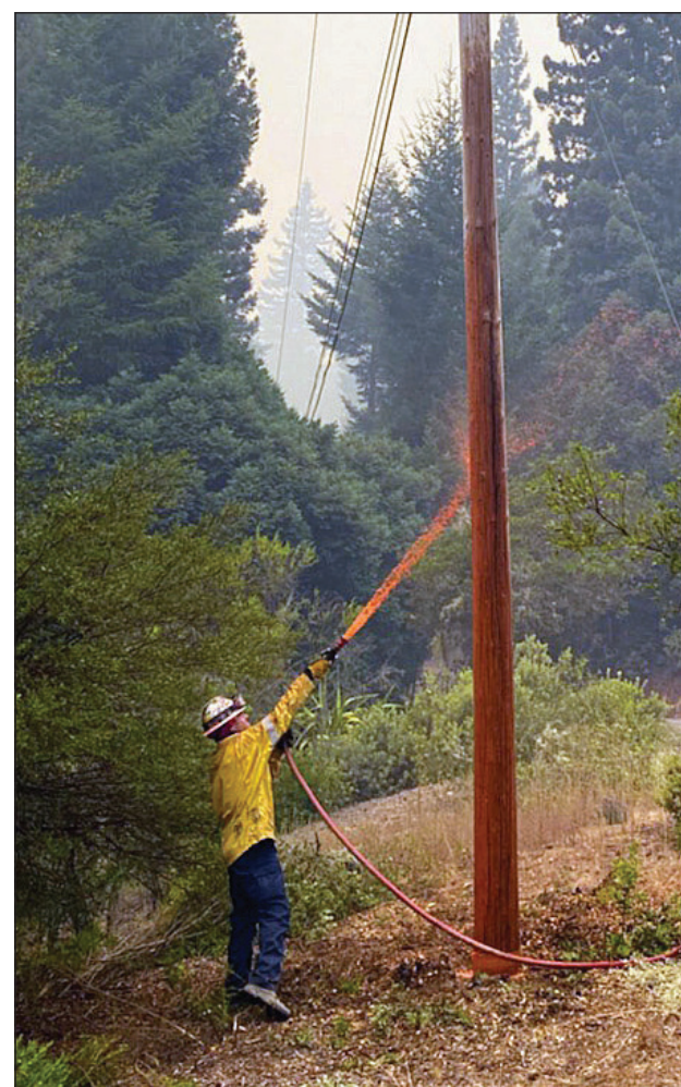
By treating poles with fire retardant, SIPT crews are able to drastically reduce the number of poles lost in fire zones.
