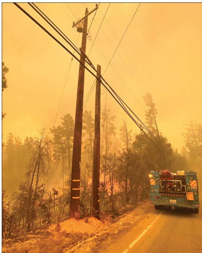
The utility pole in the background was treated with retardant by the SIPT crew, and made it through the fire.
