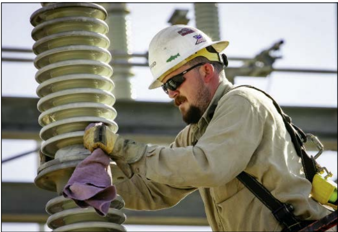
SMUD Apprentice Substation Electrician Sam Burns cleans an insulator.
