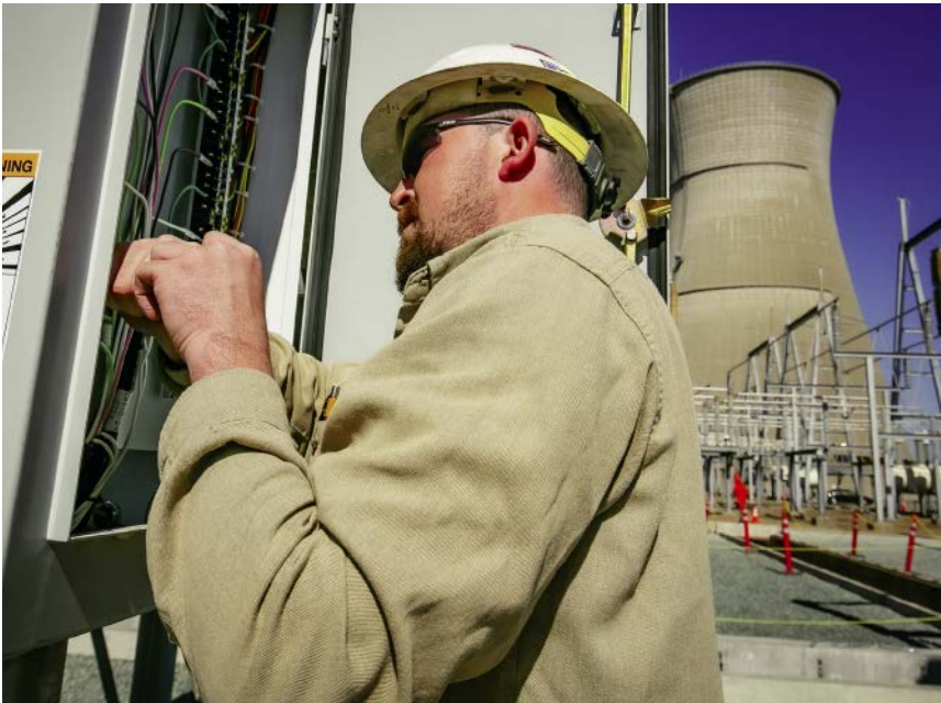
Apprentice Sam Burns working on a ct circuit in one of the new circuit breakers.
