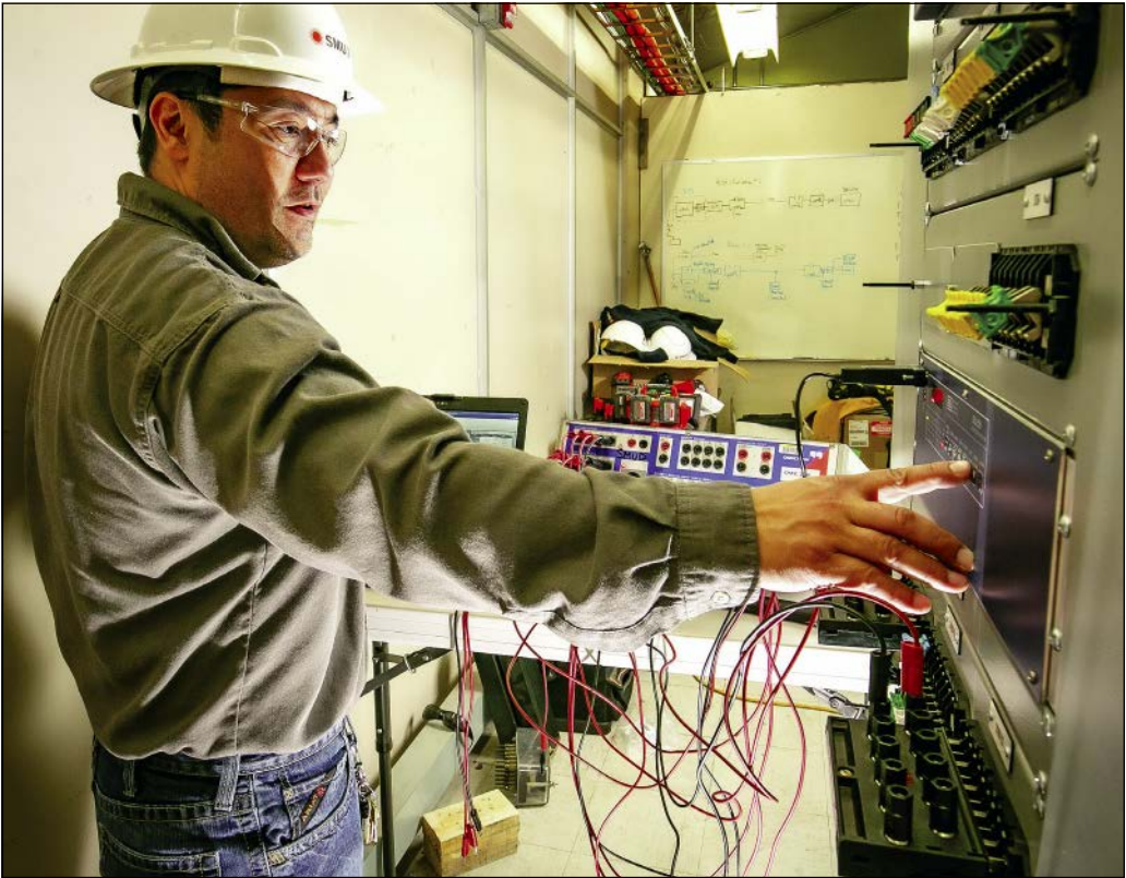
Toshi McCormick tests a breaker failure relay.
