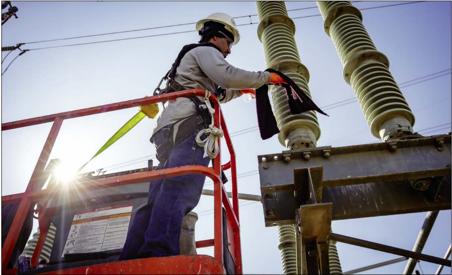
SMUD Substation Electrician Marcus Crumble cleans insulators.
