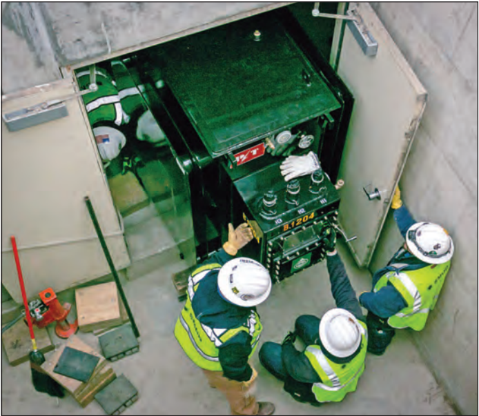
SMUD linemen move the transformer into the vault.
