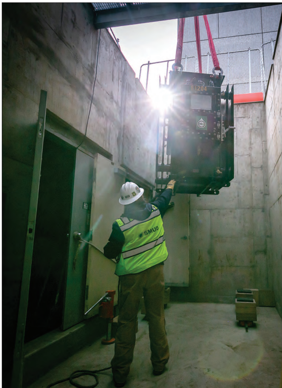
SMUD lineman Ryan Malmberg guides one of the transformers onto the skates.
