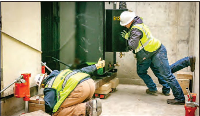
SMUD linemen move the transformer into the vault.
