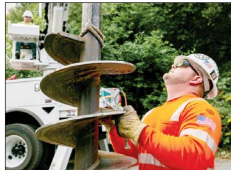
Joshua Olson works with an auger to replace poles.
