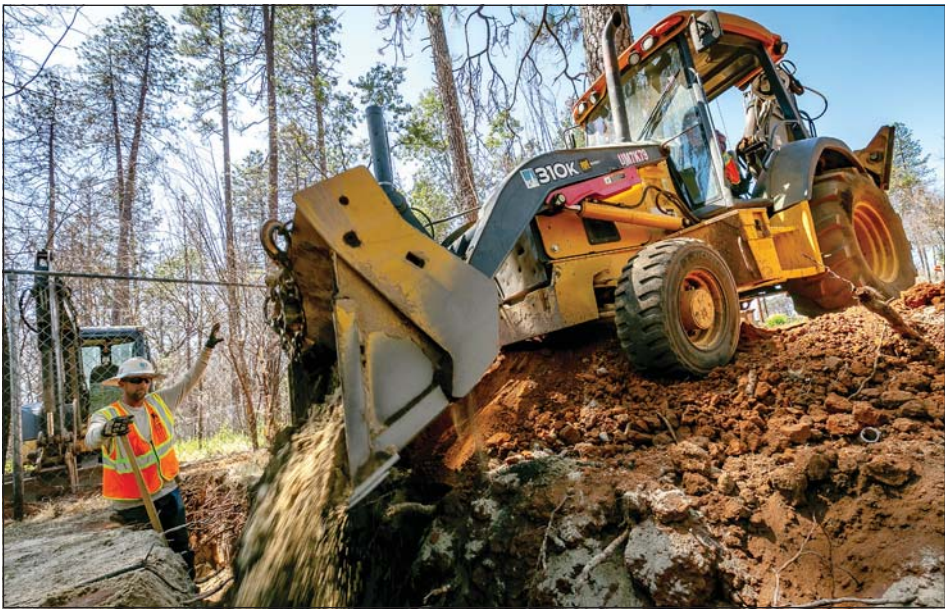
Josh Summers guides the backhoe to dump gravel into the trench.
