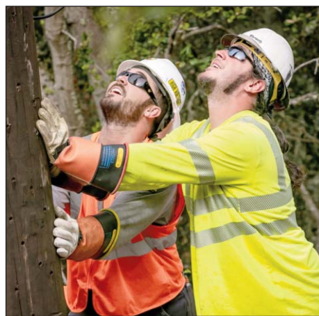
Will Warmoth, (right) and John Beckman guide a pole into the hole.
