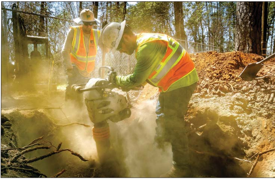
Kemmer Stephens tamps down the gravel in the trench as Josh Summers watches.
