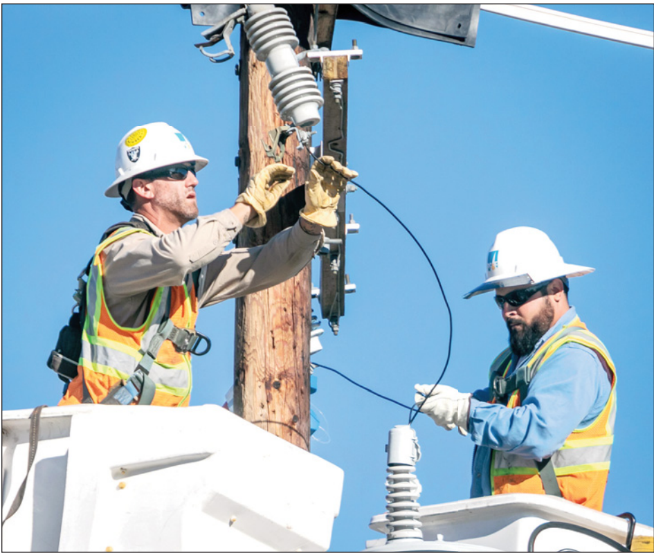
A PG&E crew replaces a transformer. Photos by John Storey
