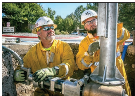
Apprentice fitter Michael Kennedy (left) and welder Troy Callahan drill into a pipe.
