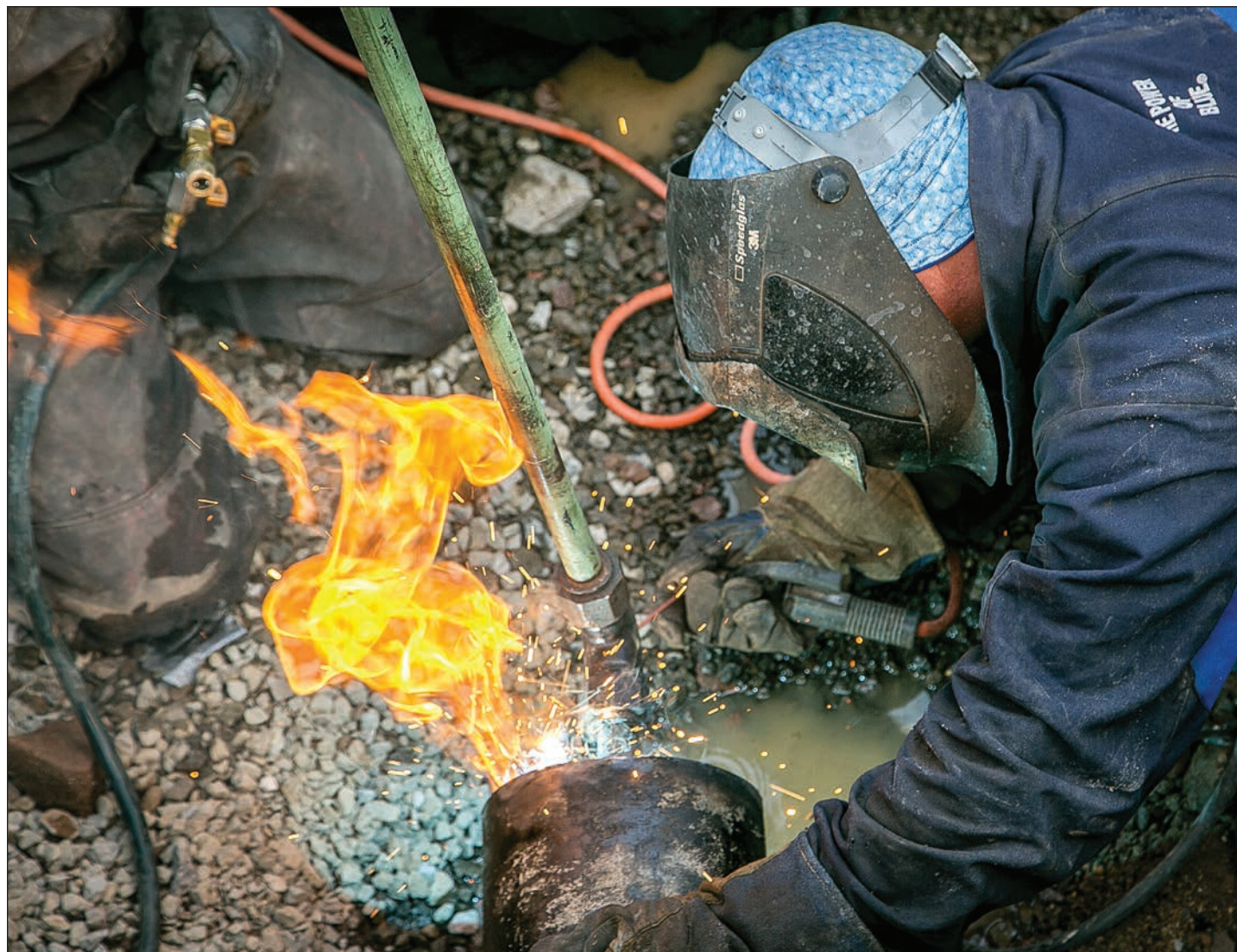
NV Energy welders Troy Callahan (left) and Richard Eisenbeiss weld a cover on a gas pipe in a neighborhood in Sparks, Nevada.
