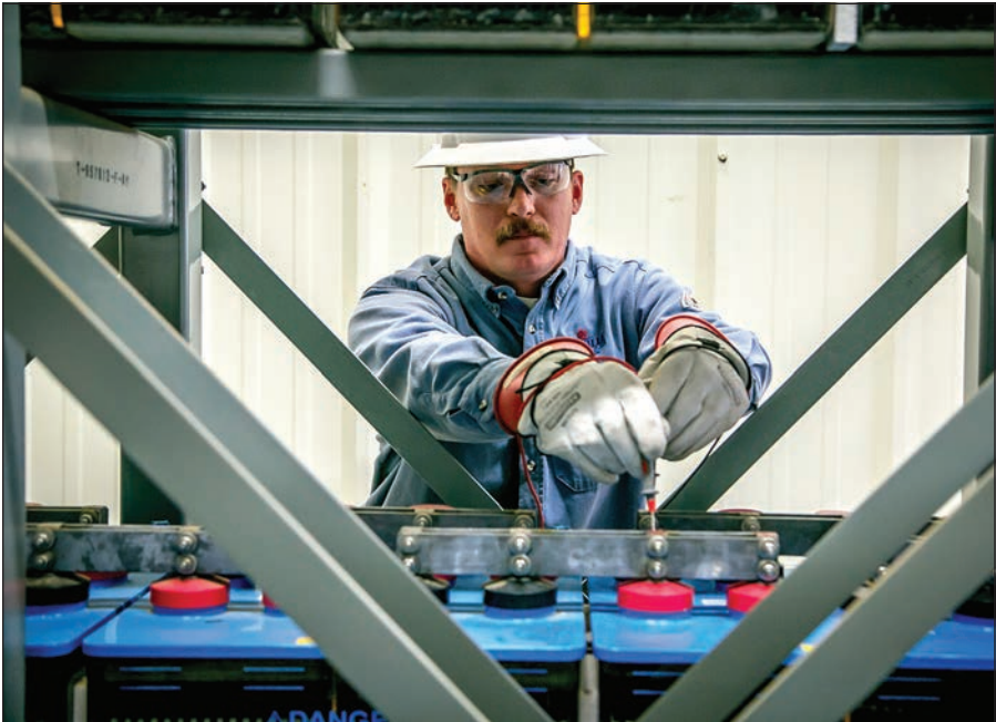
Electric Utility Technician Brett Dietz checks the back-up batteries at the power plant.
