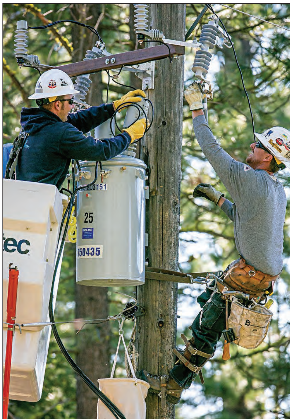
Kyle Hermansen, in the bucket, and Toak Scarlett connect the transformer leads to the cutouts.
