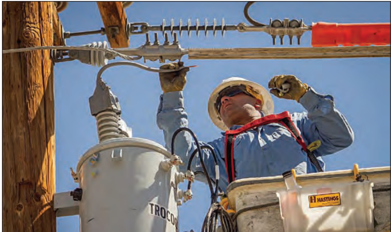
Apprentice Lineman Jared Dillard hooks up the transformer.
