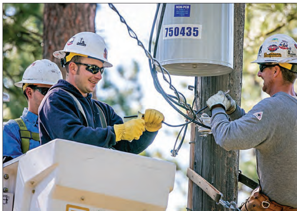
Kyle Hermansen, in the bucket, and Toak Scarlett prepare wire to reconnect a service drop.
