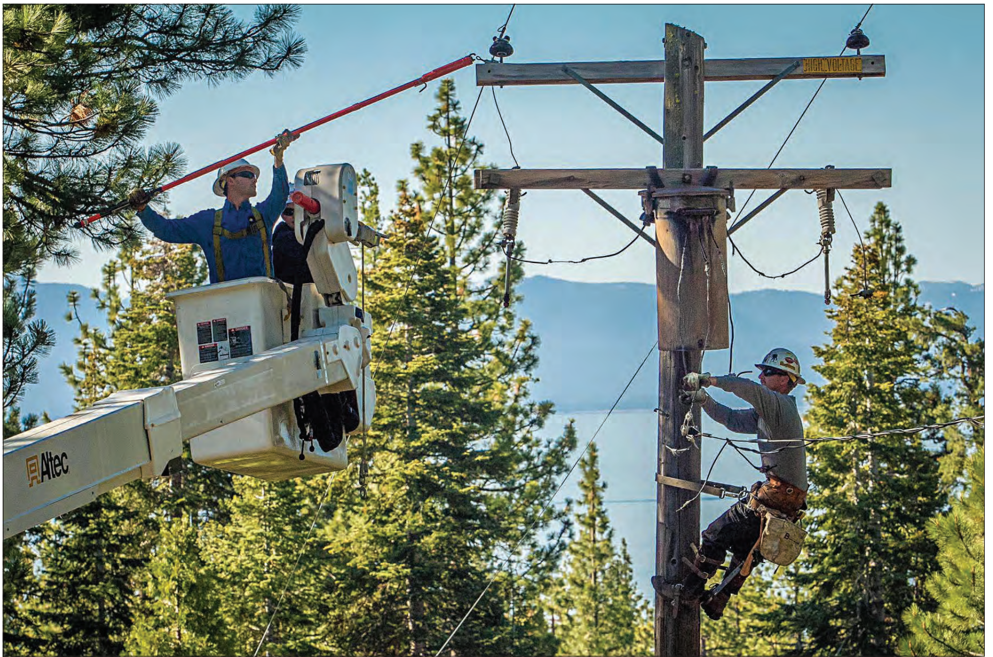
Ross Leone, left, works from the bucket and Toak Scarlett works from the pole as the crew isolates the old transformer for replacement.
