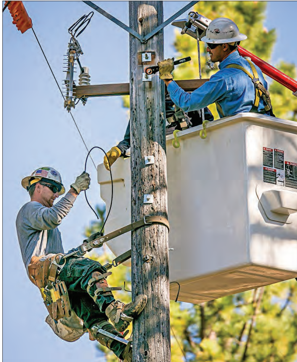
The crew mounts the equipment arm, in preparation for the transformer upgrade. Toak Scarlett is on the pole, while Ross Leone and Kyle Hermansen (behind the pole) work from the bucket.
