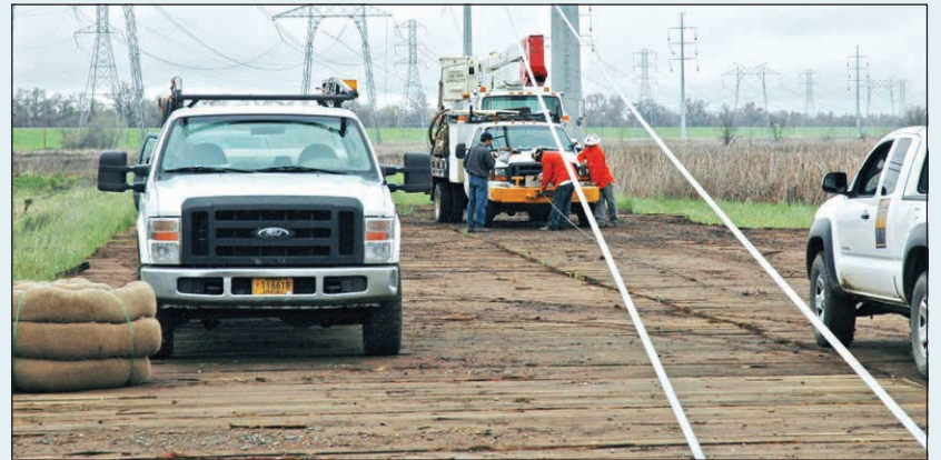
Wooden planks cushion the vehicles' impact on the land.
