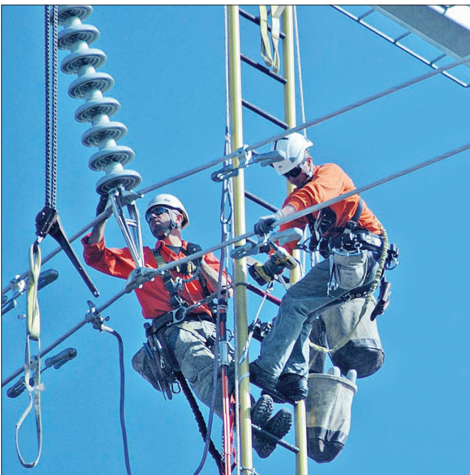
LEFT: Clipping conductor into the shoes at the base of the insulator.
