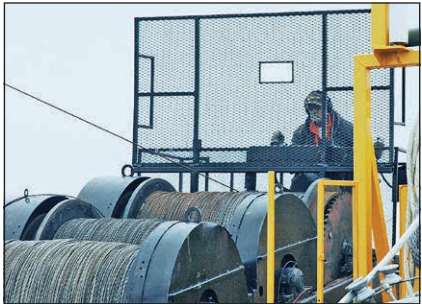
This "sockline" is used to pull in the steel cable that will be used to pull the conductor.
