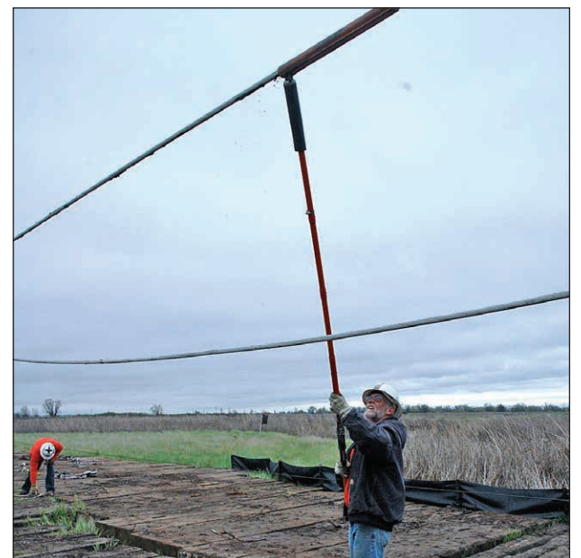
LEFT: Clipping conductor into the shoes at the base of the insulator.
