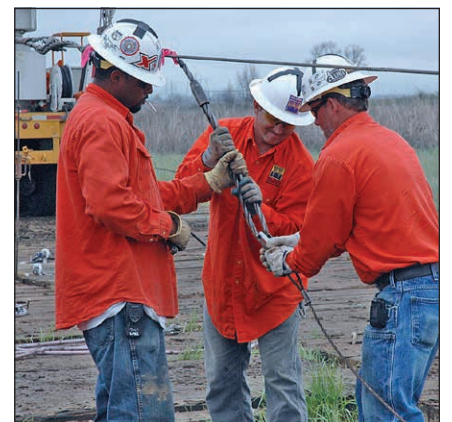
LEFT: Orange hose is used on the conductor to protect it from bumping into the pulling wire.
