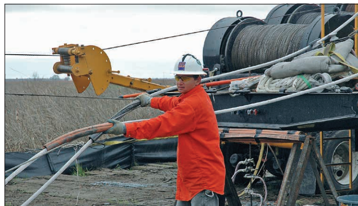
LEFT: Orange hose is used on the conductor to protect it from bumping into the pulling wire.
