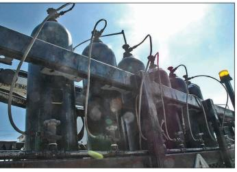
[LEFT] Nitrogen is used to blow the "pig" to the pulling end of the job, where it is attached to a cable line, which is dragged back to the end where the cable spools are located. The cable line is then attached to a "head" where all three cables come together.
