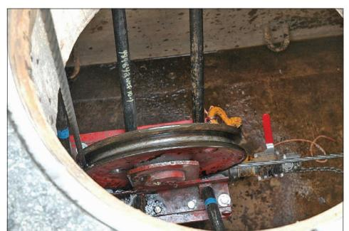
This underground wheel keeps the cable centered in the pipe during the 600-foot pull. This will be the termination point of the pull.
