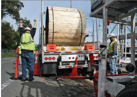
Stop right there! The cable spools have to be aligned just right. A bad angle at the front end of the pull would be amplified en route to the other end—causing the cable to bind up.
