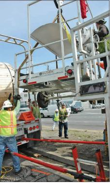
Lowering the camera trailer into place. The cable will be video-taped as it comes off the spools to document any defects.
