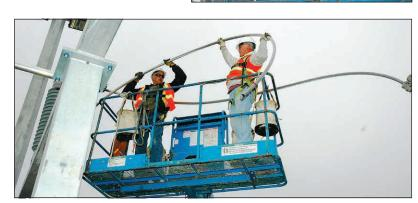
Evans and Trillo installing jumpers to 115 kv breaker.
