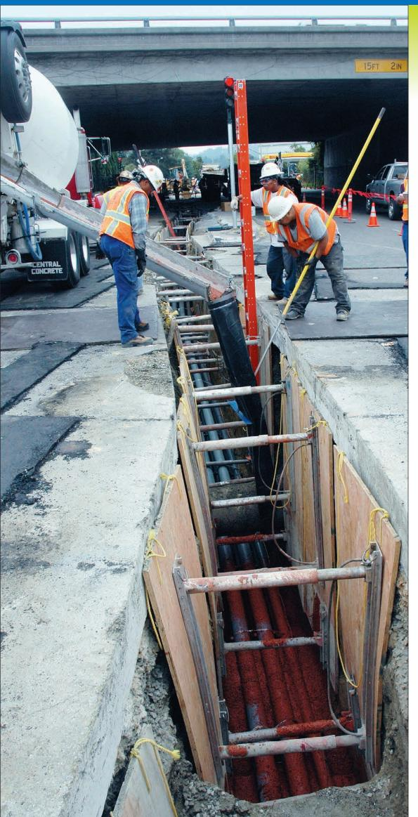
The trench is shored and the conduit laid as the job progresses up Park Blvd. in Oakland. In the distance, the excavator extends the trench under Interstate 580. Pouring a specially designed thermal cement that will help dissipate heat generated by the electricity in the cable are, from left, Technicians Daniel Wheeler, Tonisha Tizeno, and Douglas Castillo (bending down).
