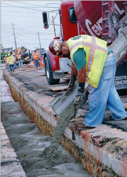
After the thermal cement is poured, the trench is topped off with thermal backfill by Foreman Alfredo Escobedo.
