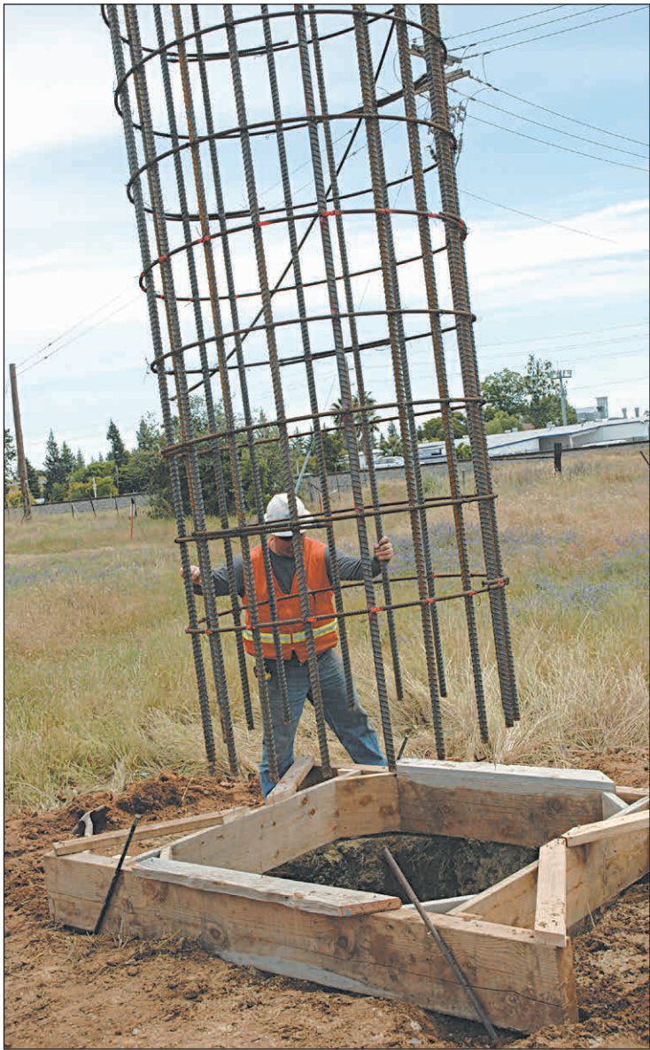
5 Positioning the rebar cage.
