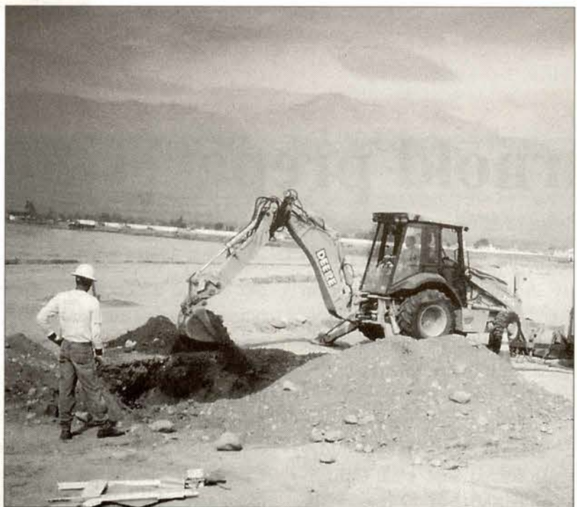
Looking for the break in the hardline.
