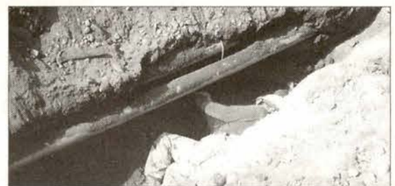
Bill Claunch cuts window in PVC to find end of hardline that snapped during a 1450-foot pull.
