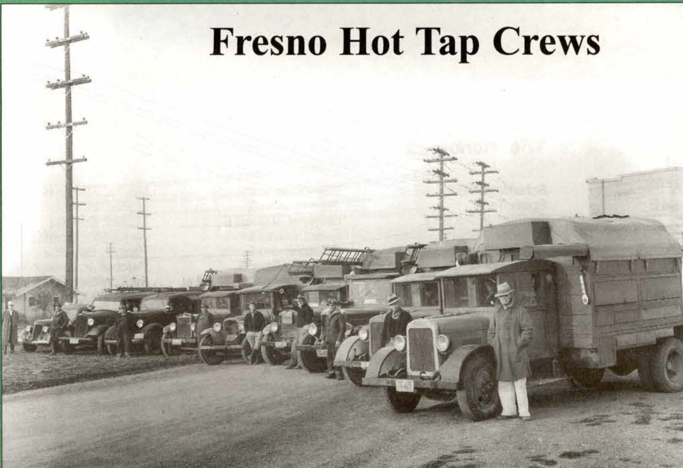
Fresno "hot tap" crews ready for work on Dec. 8, 1936, for San Joaquin Power & Light, whose service territory is now served by Pacific Gas & Electric.
